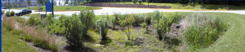
Bioinfiltration Traffic Island
