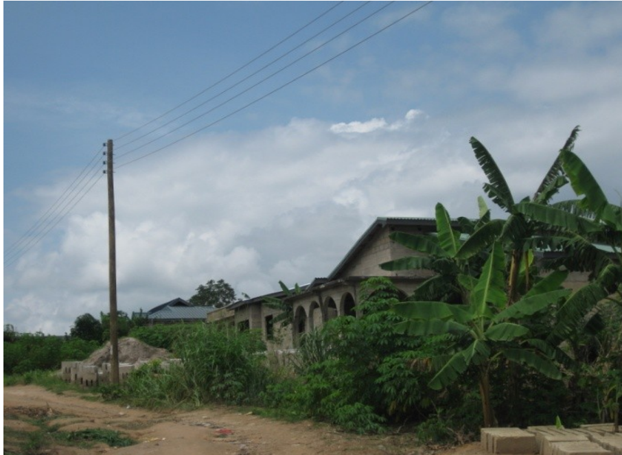
Figure 3 A residence at Oti
