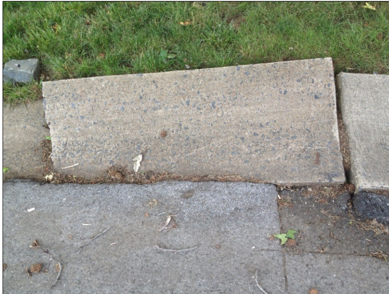
Figure 21. Dislocated Sidewalk Segments
