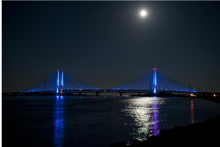
Figure 2 Elevation View of the Indian River Inlet Bridge
