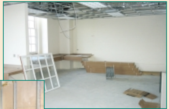
Seminar room under construction
