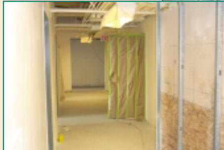
3rd floor hallway in preparation for painting
