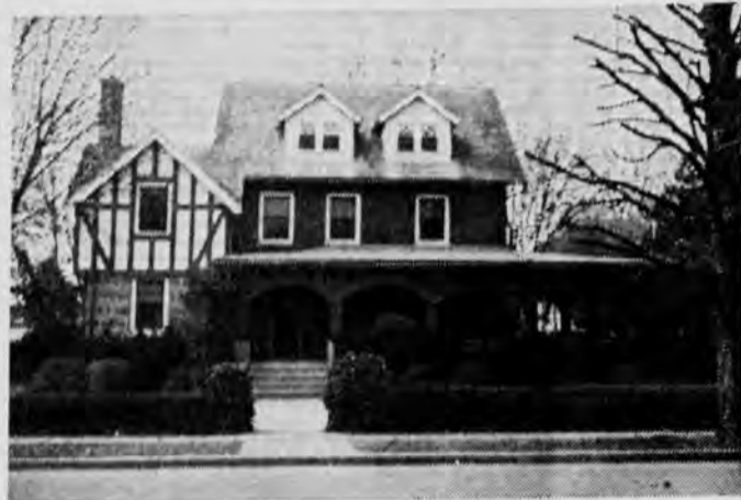
New future home of Phi Kappa Tau fraternity at 186 S. College Avenue, which will be occupied soon after completion of rejuvenation.
