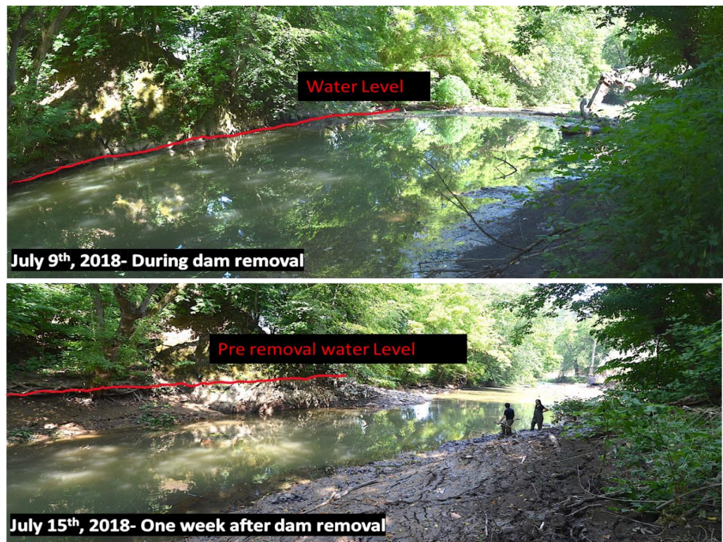
Figure 3.1: Stream water level before and after dam removal at the site of the Krady milldam
