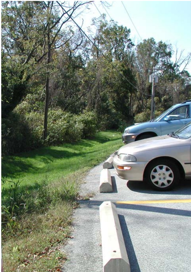
Figure 6: Image of Clayton Hall Stormwater Swale Running along the Alpha Sigma Alpha Parking Lot.
