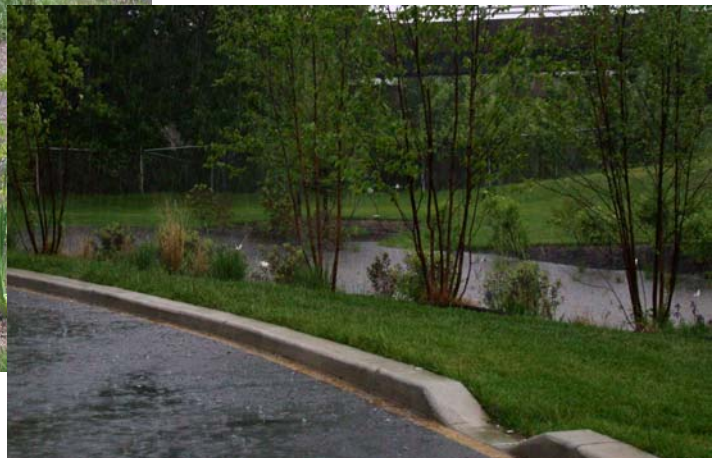
Figure 4: Dickinson Bioretention Basin in the Rain
