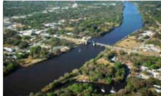
Hendry-Glades County Bridge
