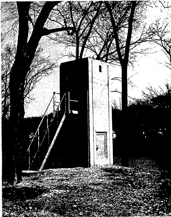
Figure 8.—Reinforced-concrete well and shelter. Note clean-out door.
