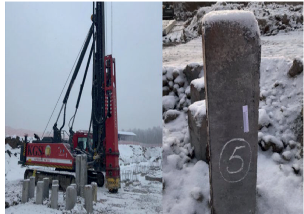
Figure 3. a) Junttan PM-25HD piling rig in Nur-Sultan city, b) test pile
