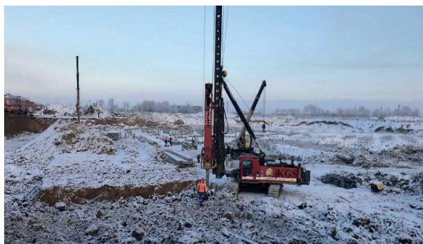
Figure 4. Junttan PM-25HD piling rig in Petropavlovsk
