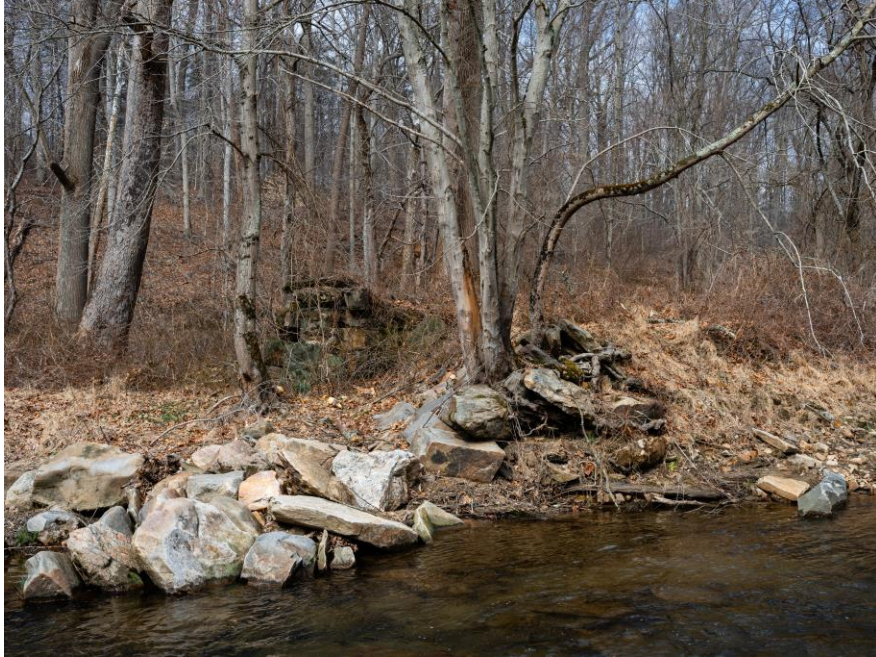
Figure A5: Dam remnants at the Big Elk Creek, downstream site. Note remnants of retaining wall in the background.
