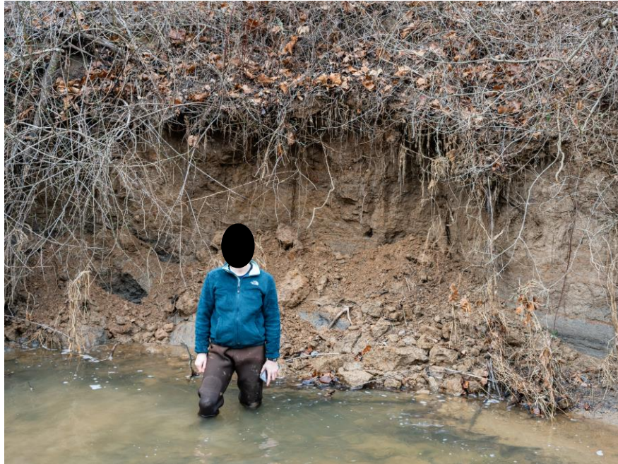
Figure A7: Stream bank erosion at the Big Elk Creek, downstream site following the February 2018 storm events.
