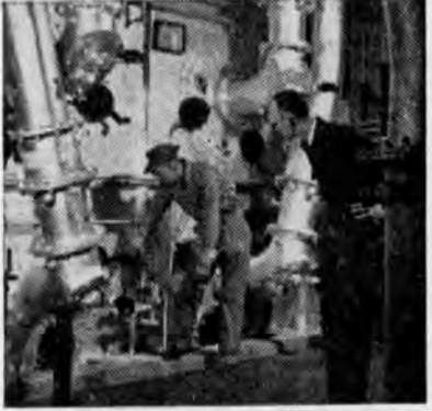
A FIREMAN adjusts louvers for the proper combustion of pulverized coal. Blown into furnace through pipes, it burns at 2500°F.
