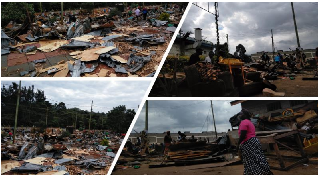
Image 16: Sites of demolition in Kibera on June 21, 2018
