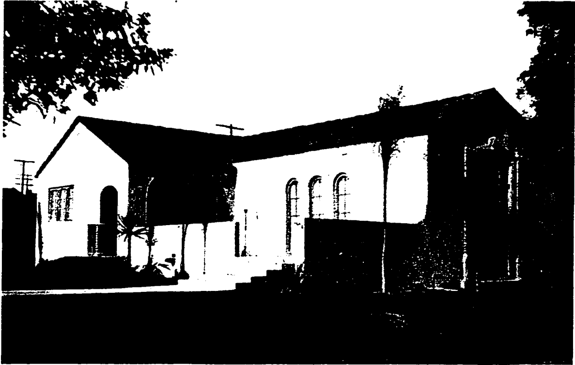
Figure 1. Small residence in Los Angeles. R. Newcomb, The Spanish House for America , p. 38.
