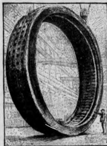
A casting for one of the huge water-wheel driven generators installed in the Mississippi River Power Company's plant at Keokuk. This installation will ultimately consist of thirty of these machines, giving a total capacity of 216,000 kilowatts (300,000 horse-power). It is the largest hydro-electric development in the world. The General Electric Company builds generators for water-wheel drive in sizes ranging from 27½ to 25,500 kilowatts and the aggregate capacity of G-E units now in successful operation is in excess of four million horse-power.
