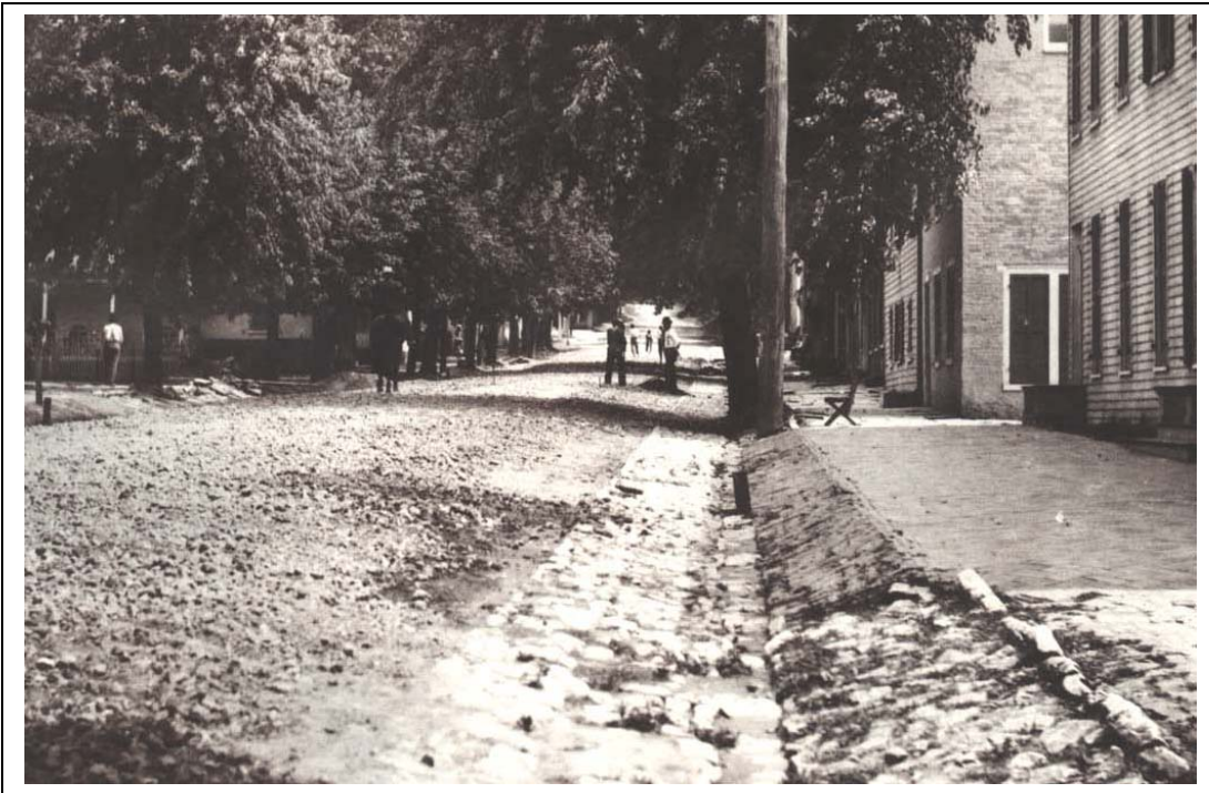
Macadam surfaced road, showing stone gutter, curb, and sidewalk. Westminster, Maryland, date unknown Source: ARBA Pictorial History
