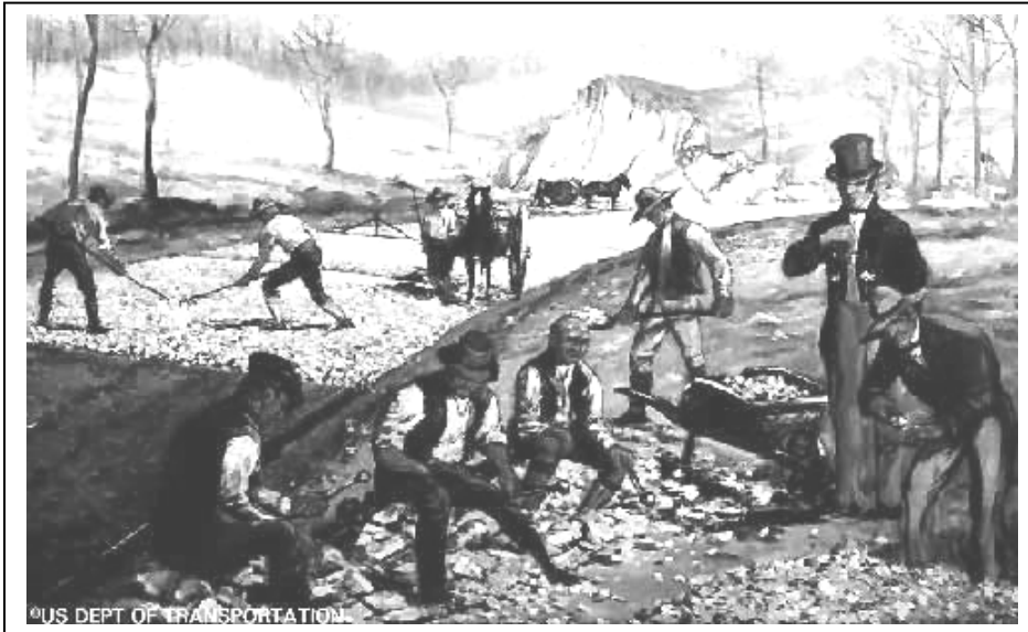
Constructing a Macadam road
