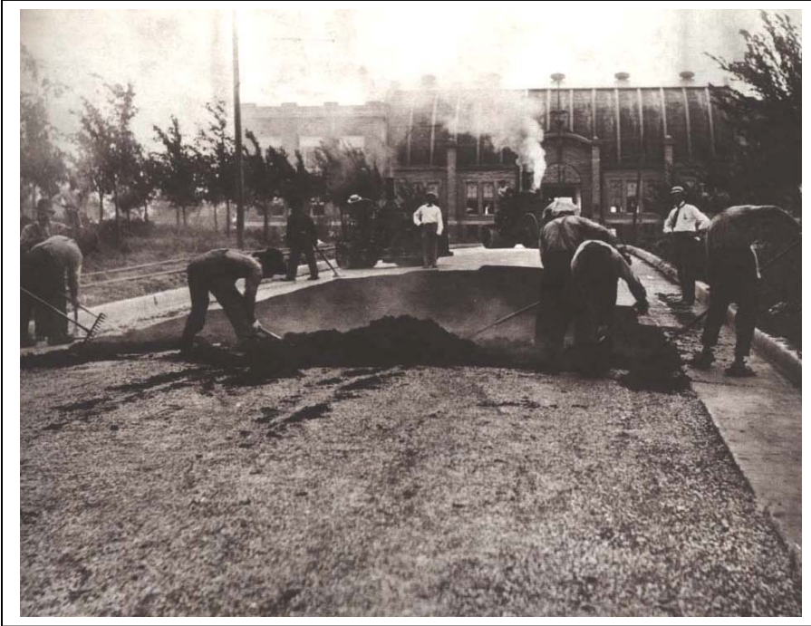
Laying asphalt paving, location unknown, ca. 1900-1915 Source: ARBA Pictorial History
