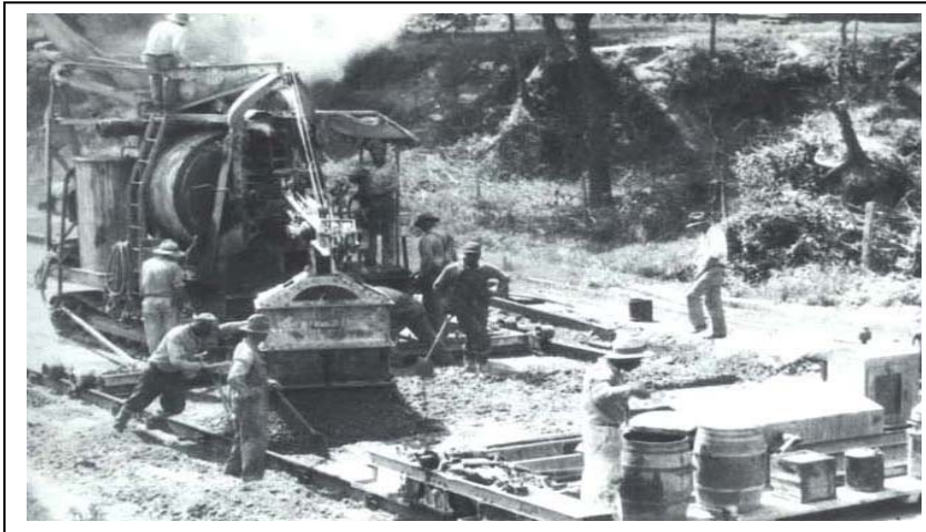
Constructing U.S. 40, Ohio, 1940
