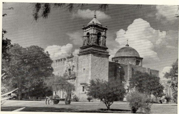
FIG. 3. Mission Church of San José, San Antonio, Texas. [Texas Highway Dept.]
