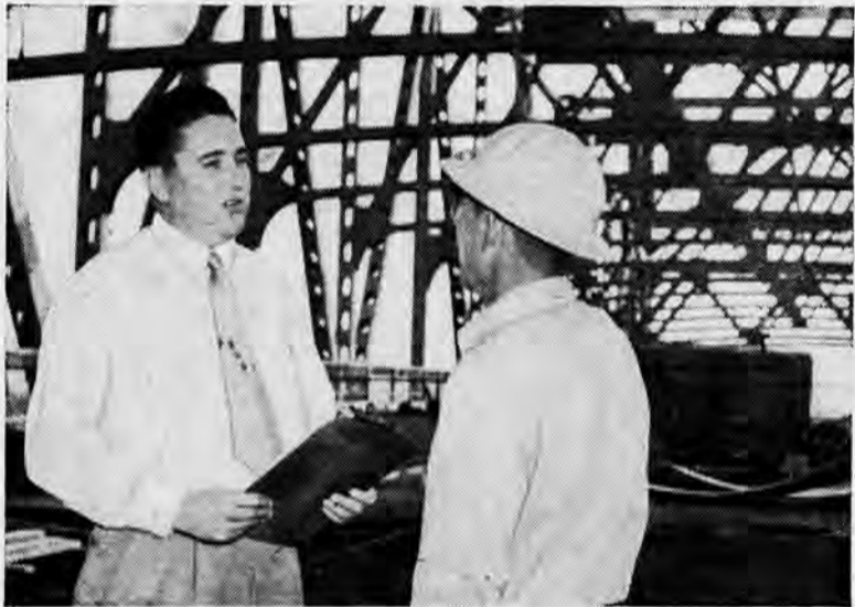
Bill Rhode (left) at the site of New Orleans' new Claiborne Street Industrial Canal Bridge.
