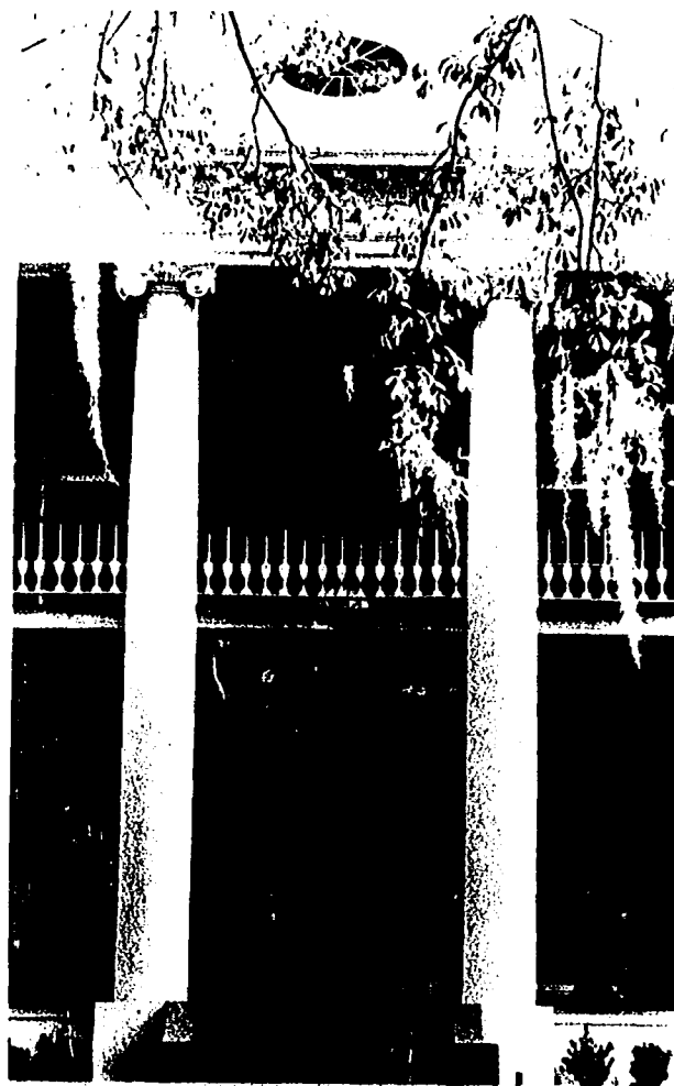
Figure 9. Detail of facade, central section, Auburn.
