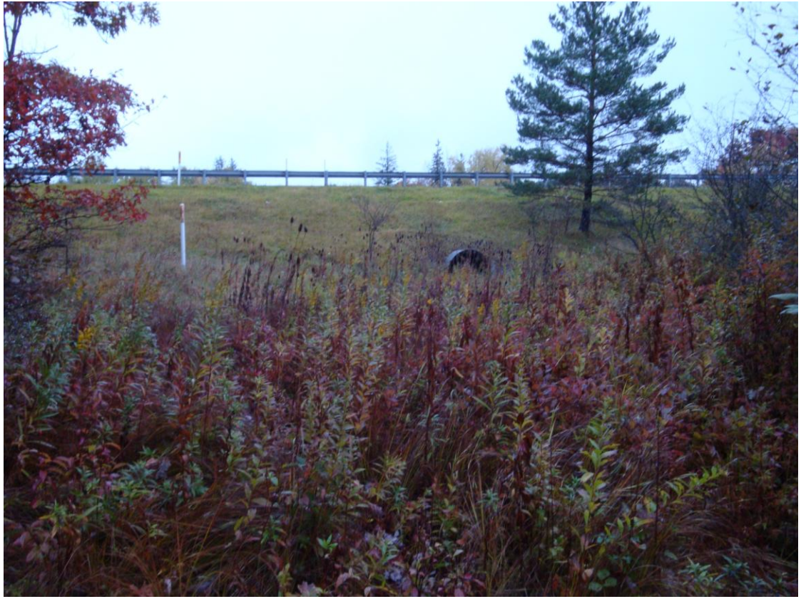
Figure 2. Rescue squad site showing the gas line disturbance and the highly traveled highway adjacent to this wetland. This photo was taken in September 2009.
