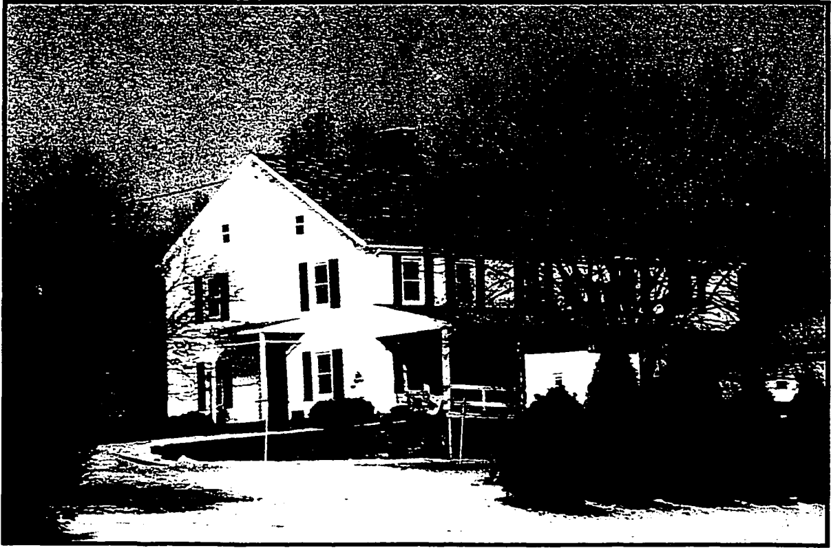
Figure 4. The Peter Good House, circa 1790. View facing northwest. The log Peter Good house originally stood only one story high. A kitchen was added to the northern gable end and the house raised to two stories in the first decades of the nineteenth century. In the twentieth century, the kitchen was raised and the entire structure placed under one roof.
