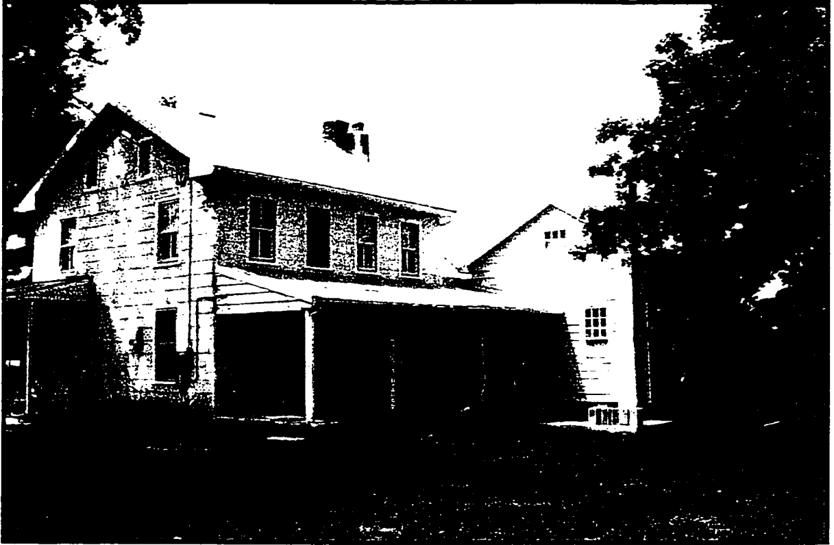
Figure 29. Example of Wood-Framed Construction and the Pennsylvania Farmhouse Type in Manchester Township. Common on the landscape, log and wood-framed Pennsylvania farmhouses were constructed in the last half of the nineteenth century and first half of the twentieth century.
