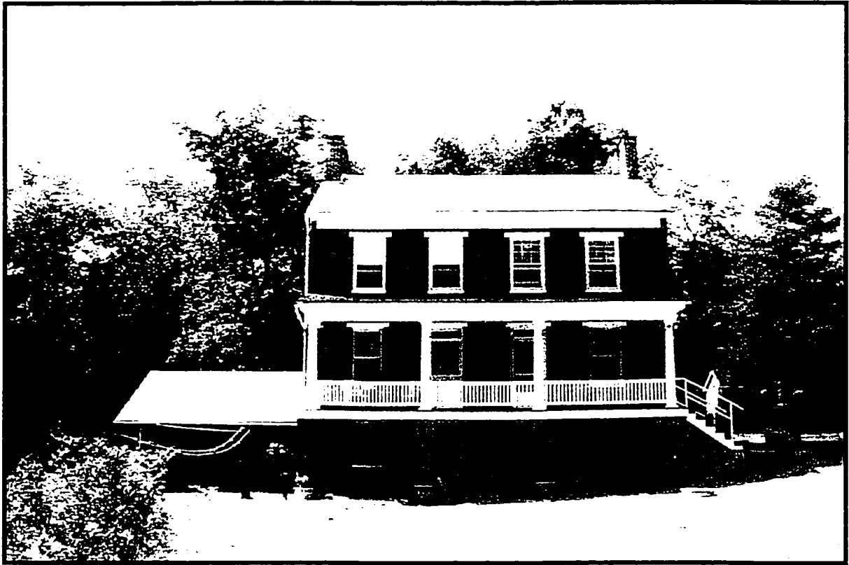
Figure 30. The Abraham Croll House, circa 1840. View facing west. The Abraham Croll house contains several hallmarks of the Pennsylvania farmhouse type: a banked cellar, symmetrical four-bay fenestration, large domestic production space, double front doors and simple exterior architectural ornament.
