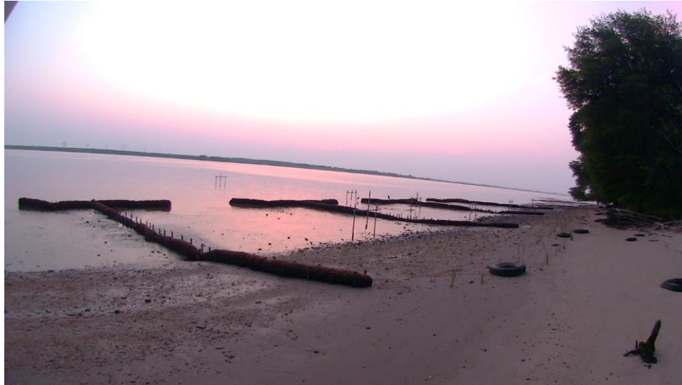
Figure 5. Live stream-captured image of final installation and sensor array.
