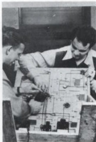
Testing electrical currents on this wiring board, 1947 electrical engineers participate in a lab project.
