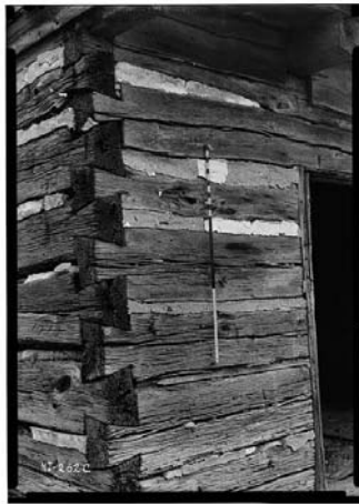
Figure 2.5a Detail, corner joinery from Mench-Reall Log Cabin (demolished), Friesburg, Salem County, NJ. Photograph by Nathaniel R. Ewan, May 9, 1936. Library of Congress, Prints and Photographs Division, HABS, reproduction number HABS NJ, 17-FRIBU.V,1—2.
