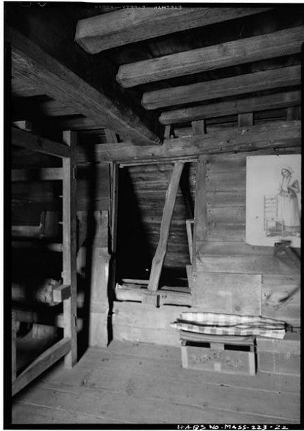
Figure 2.9a Detail of beam ends and joists, west room north elevation, second floor, Jonathan Fairbanks House, 511 East Street, Dedham, Norfolk County, MA, ca. 1636 and later. Photo by Thomas T. Waterman, June 1936. Library of Congress Prints and Photographs Division, HABS, reproduction number: HABS MASS,11-DED,1—27
