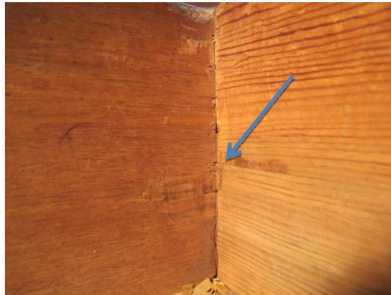
Figures 4.33 Detail, Figure 4.20. Chest of drawers made by William Beakes III. View of saw kerfs, front of smaller drawer seen from interior. Courtesy Rocky Hill Collection. Photo by author.
