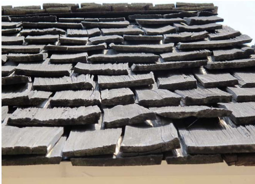
Figure 3.15 Roofing shingles, detail of Figure 3.14 (likely replaced), 2014. Photo by author.
