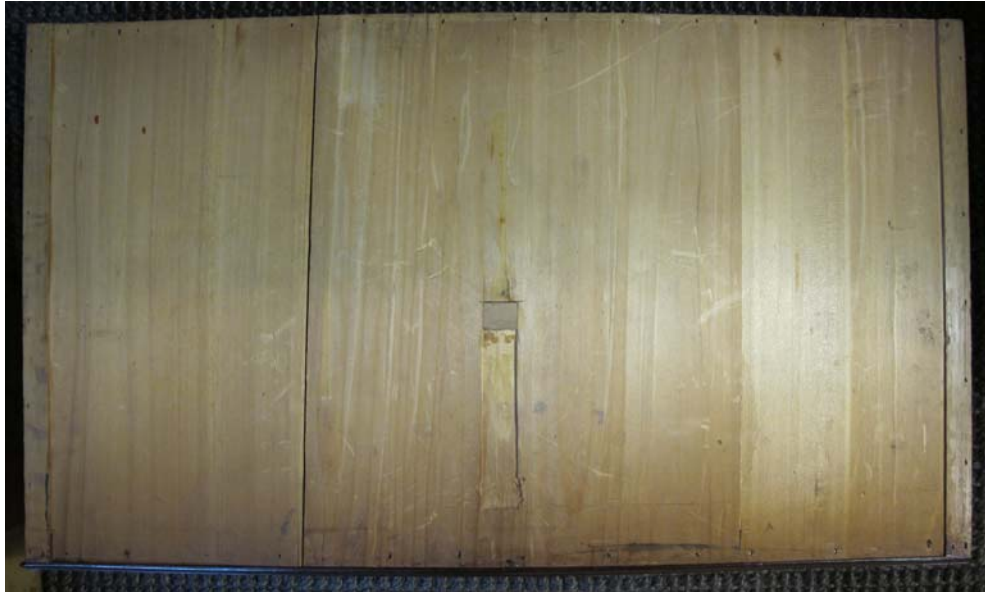
Figure 4.51 Detail, Figure 4.40. View of drawer underside illustrating regular nailing patterns. Chest on chest, dated 12 mo 1738/9. Courtesy private collection. Photo by author.
