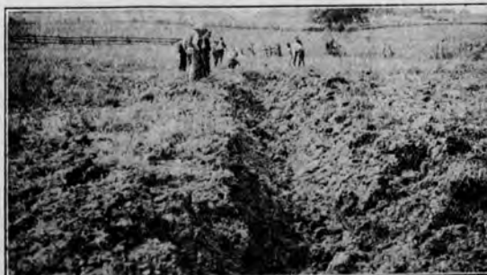
Ditching with explosives demonstration on farm of John F. Brackin, of Marshallton. Under many conditions an economical method of drainage.
