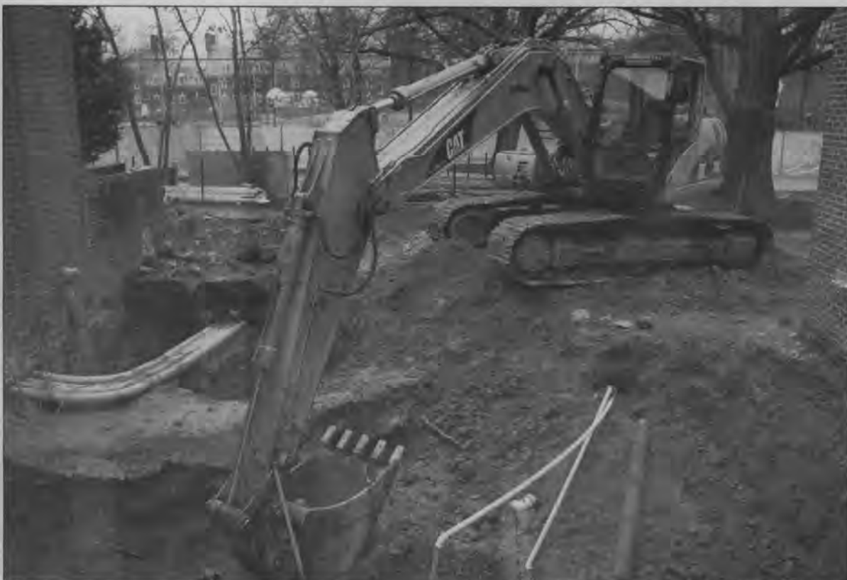
Workers are preparing to replace and enlarge a 30-year-old steam pipe near Perkins Student Center that provides heat and hot water to all of East Campus.
