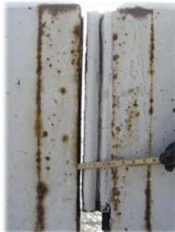
Figure 1.2 Compression Set in Bridge Parapet Joint Gland
