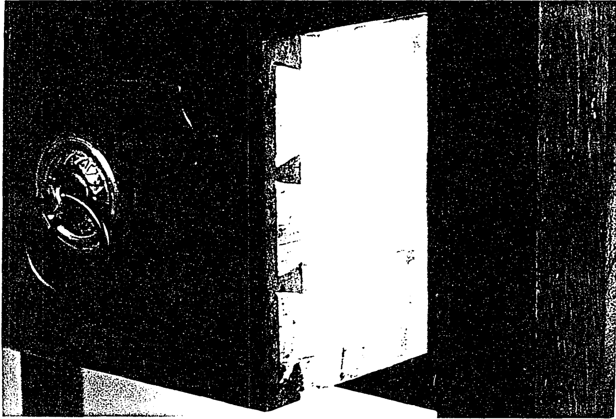
Figure 4.12 Detail of Kersh end table drawer showing commercial stamped-metal pull. Owner Charles Lenford Kersh, Harrisonburg.
