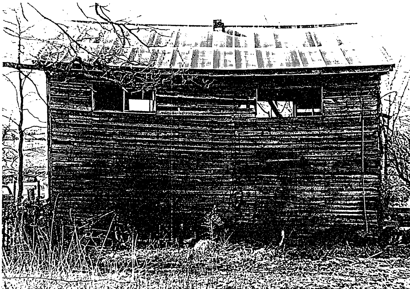
Figure 2.7 North wall of Kersh shop showing "hinged" effect of lapped construction. Kersh collection, MAFC.
