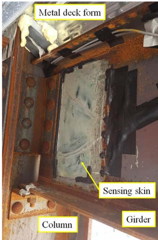
Figure 4.11: Sensing skin installed in the BPI Building
