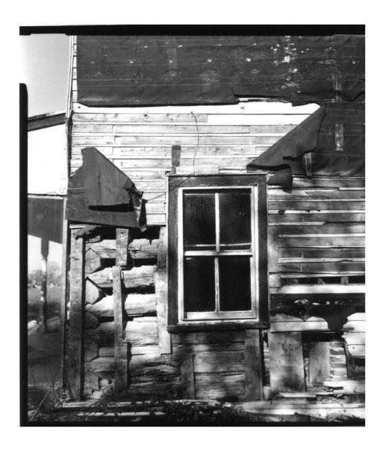
Figure 37: John Barber House, detail of the log construction on east elevation of Period I section.
