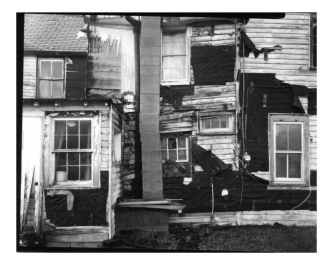
Figure 36: John Barber House, detail of the north elevation showing concrete block chimneystack and juncture of two rear additions.
