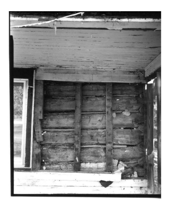
Figure 38: John Barber House, detail of the log construction on south elevation of Period I section.
