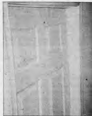
This bowed door in Danielle Harris' Riverwalk home does not meet the doorjamb even when completely closed.
