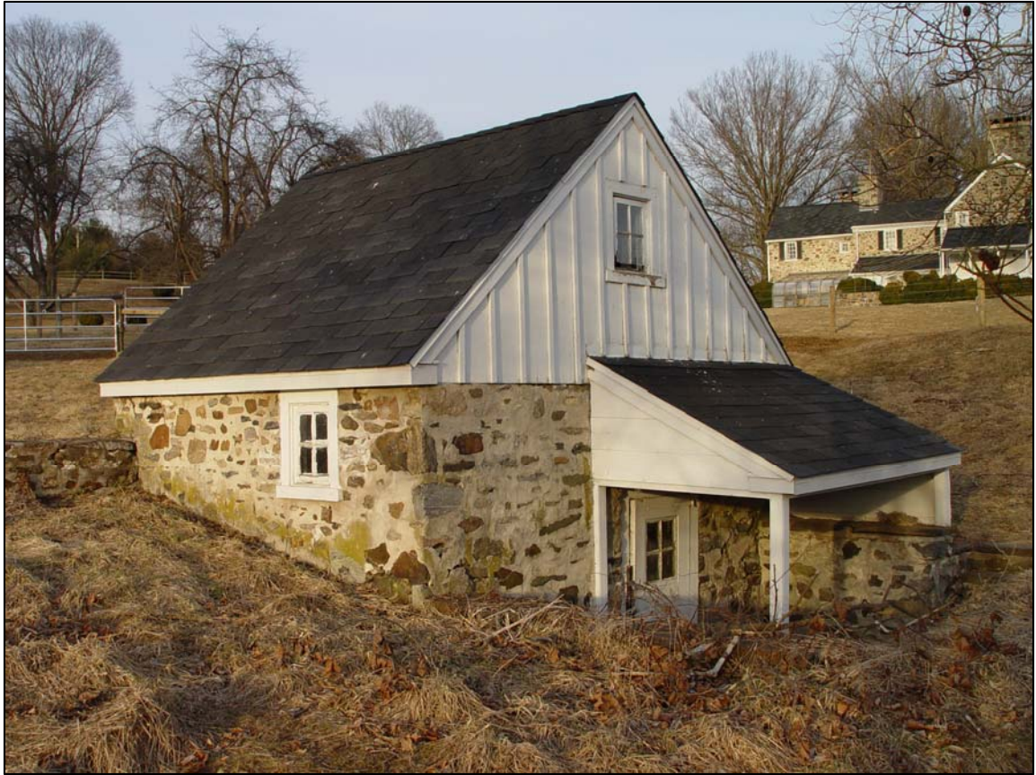
Figure 1 An example of a typical springhouse structure consisting of a stone foundation and wooden roof enclosing a spring. This springhouse was partially built into the ground, a design common among springhouses.
