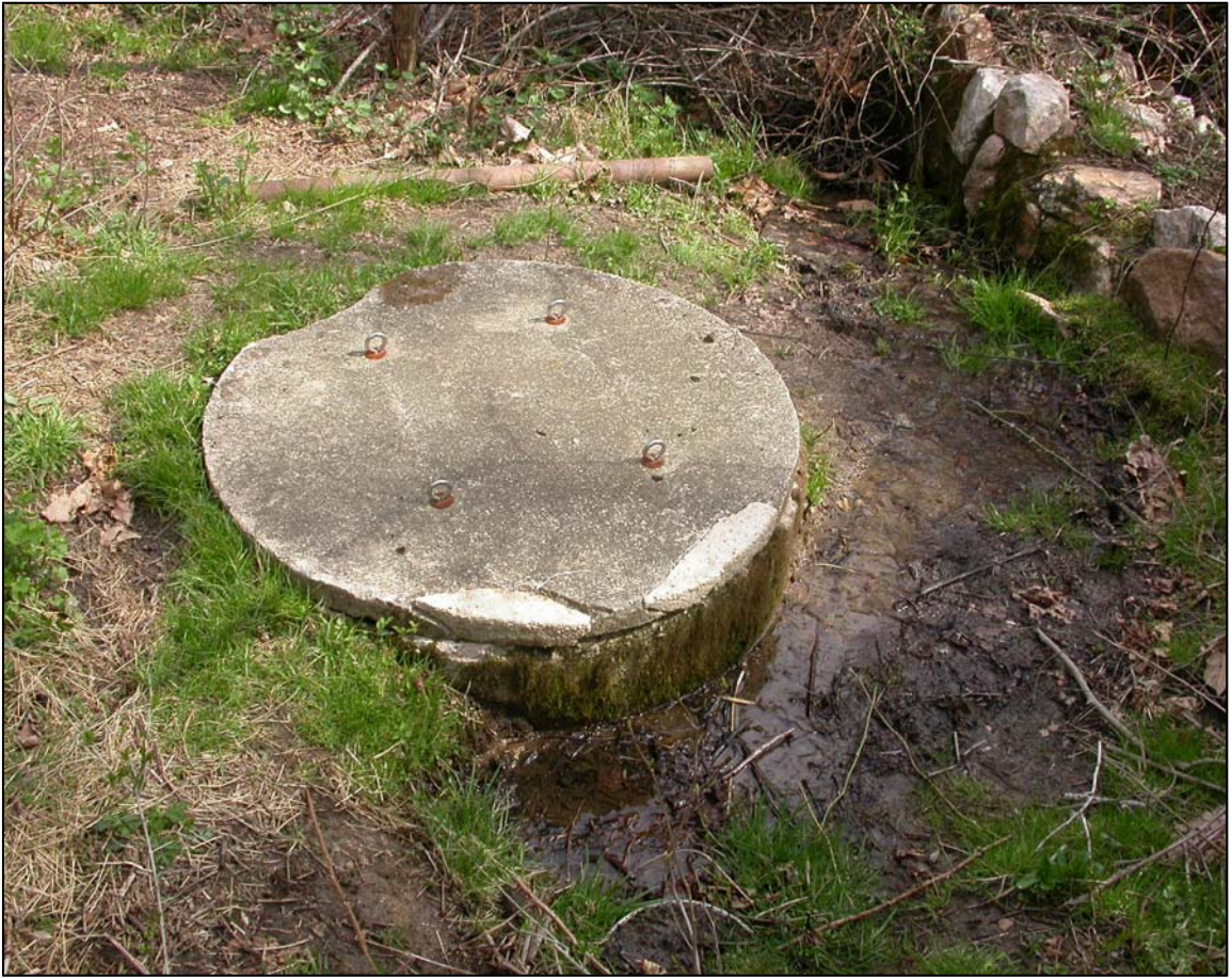
Figure 4 An example of a cement cistern or springbox capping a springhead.
