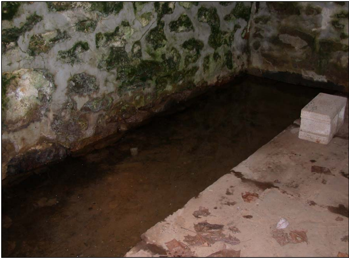
Figure 2 An example of a water compartment containing ground water near the effluence of a spring within a springhouse.
