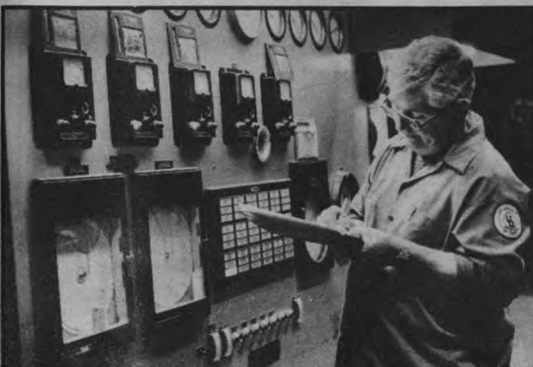
"WE PROVIDE the heat and air conditioning for central campus -- between 33 and thirty-seven buildings," said Hank Kraszewski, making his hourly check of the boilerroom machinery. At the coldest time of this year, they used over 800 gallons of oil an hour to pump 93,000 pounds of steam for heat.
