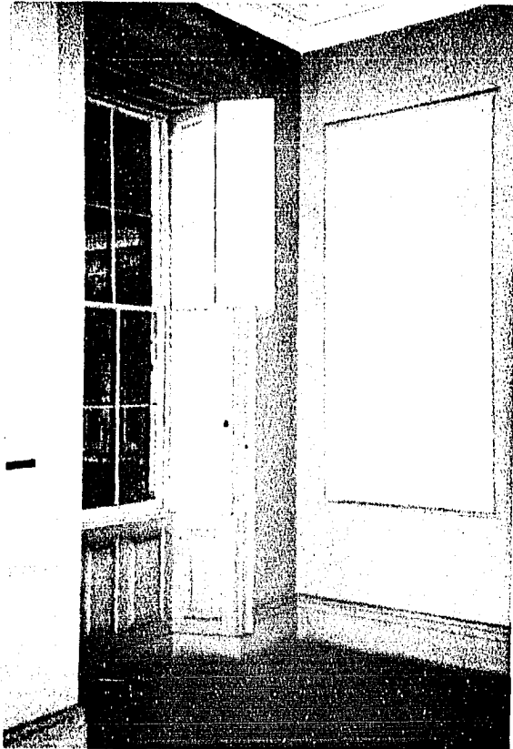
9. Corner of the Southwest Parlor of The Highlands Showing Original Paneled Interior Shutters
