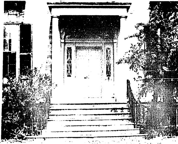
14a. Entrance Door at The Highlands, Exterior
