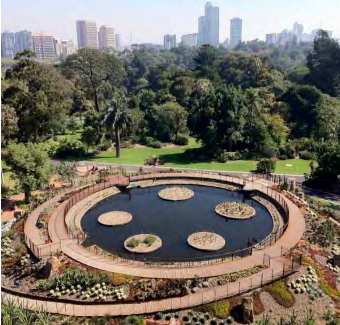
Figure 5.3 Guilfoyle's Volcano, part of the Melbourne Garden's stormwater harvesting project. Note the floating wetlands, a practical and attractive feature of the scheme. (Source: RBG Victoria).
