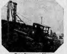
POLE SETTER AT WORK
