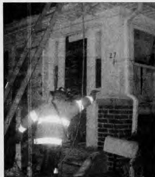
THE REVIEW/Christian Jackson The fire at 27 Lovett Ave. on Jan. 25 was caused by a kerosene heater left unattended, according to officials.
