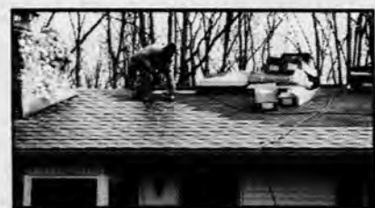
We now have metal roofing
