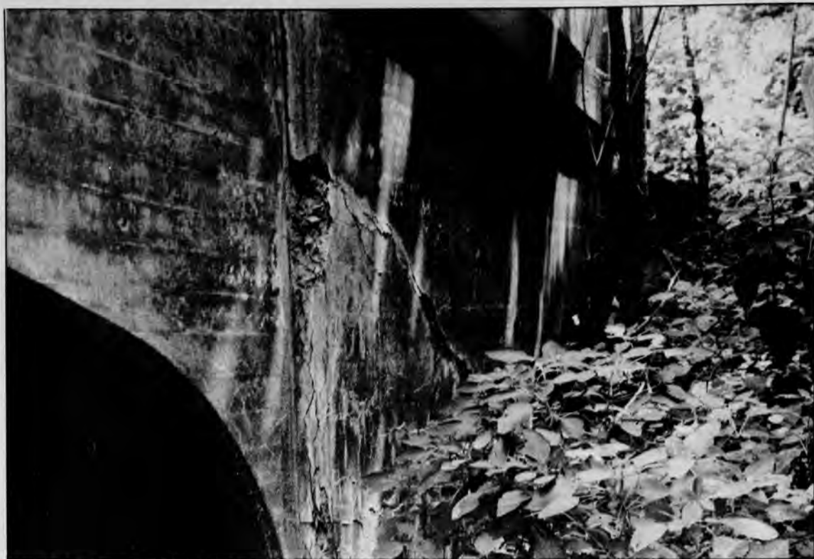
The state has placed a weight limit on the Nottingham Road bridge, which spans Christina Creek near Casho Mill Road.
