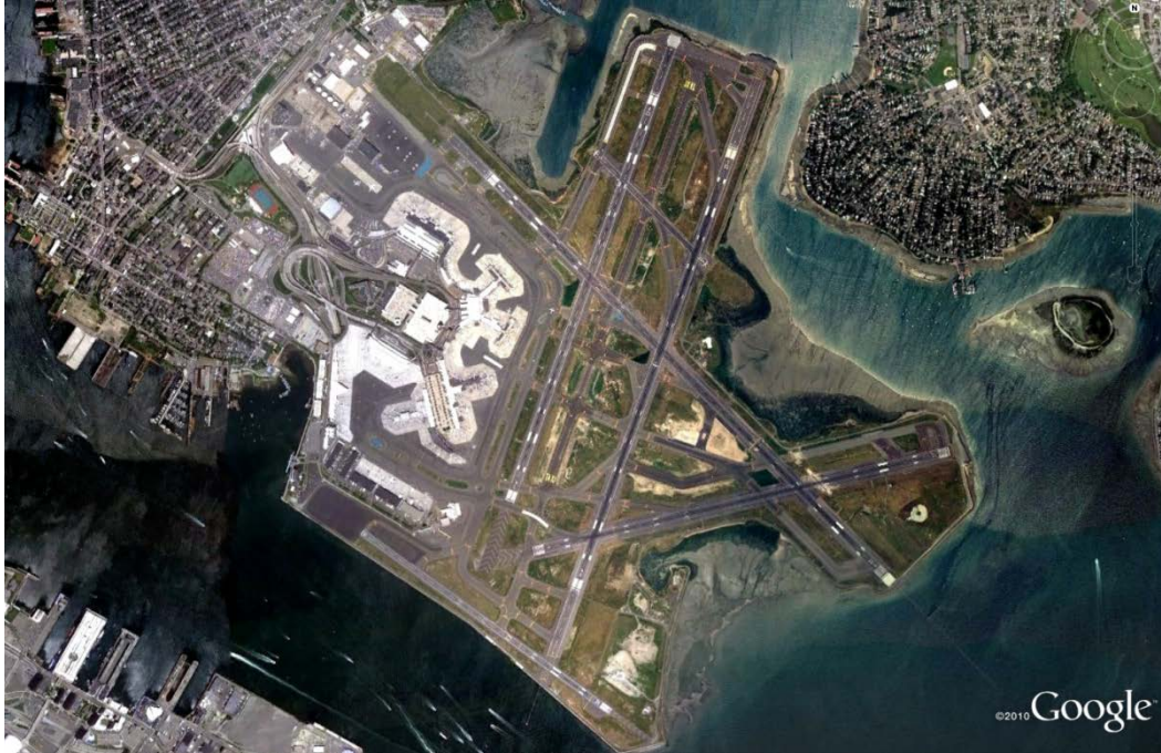
Figure 3.2: Ariel View of Boston Logan International Airport (©2012 Google, ©2012 Europa Technologies)
