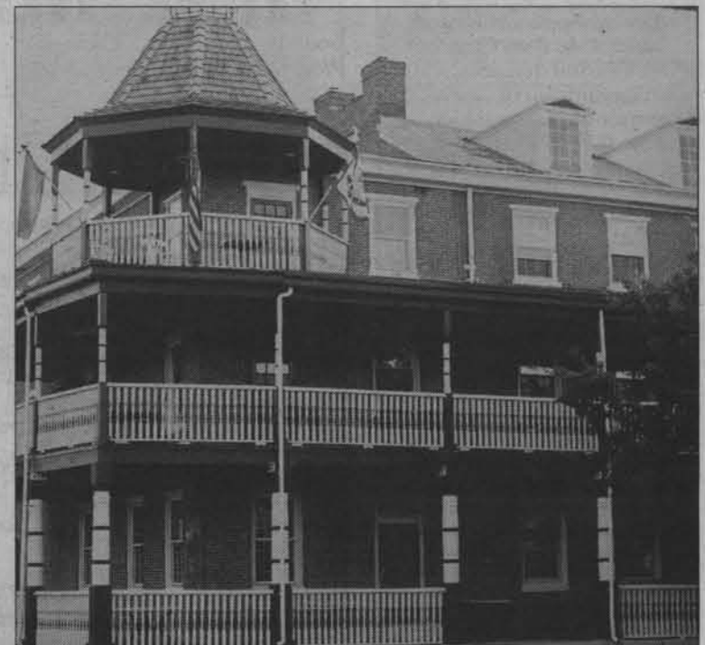
The Deer Park Tavern, 108 W. Main St., has received the "A Better Newark Award" by Newark's Conservation Advisory Commission. The Deer Park Tavern was chosen because of the extensive renovations made to the interior and exterior of the building. The Deer Park Tavern is listed on the National Register of Historic Places.
