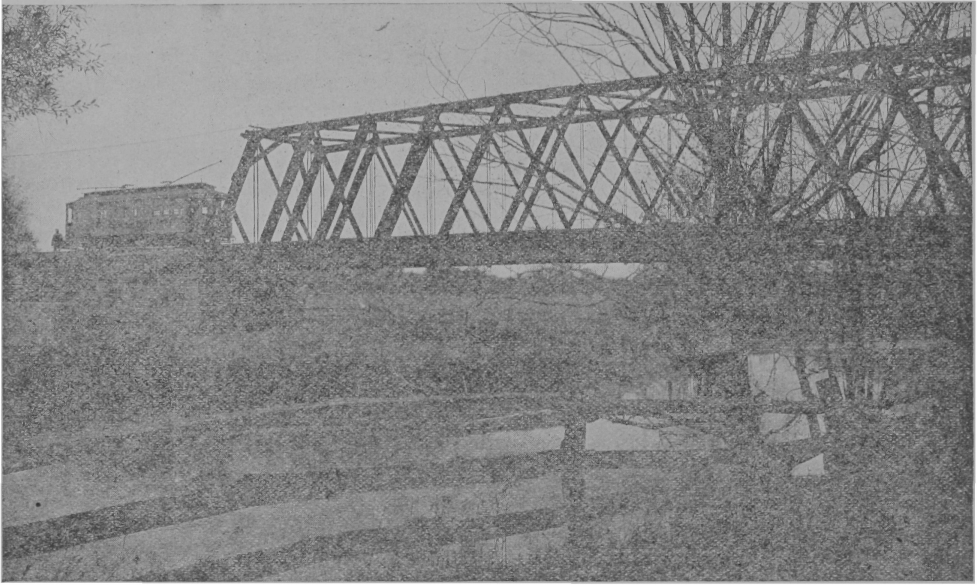
BRIDGE ACROSS THE CONESTOGA NEAR BLUE BALL
