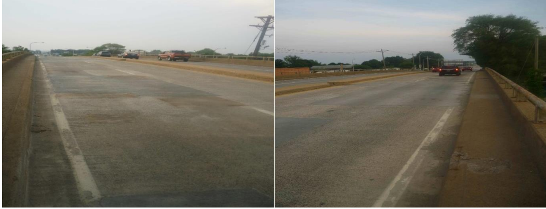
Figure 2.12: Bridge deck from both sides of approaching traffic.
