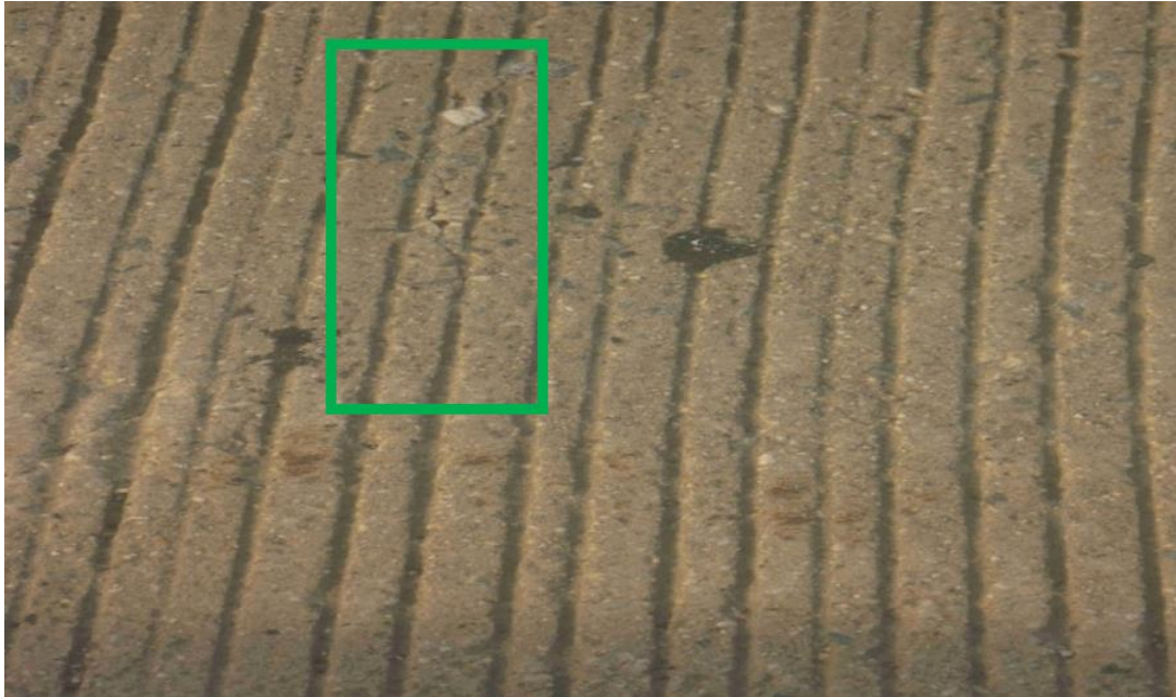
Figure 2.10: Example of shrinkage and creep cracks.
