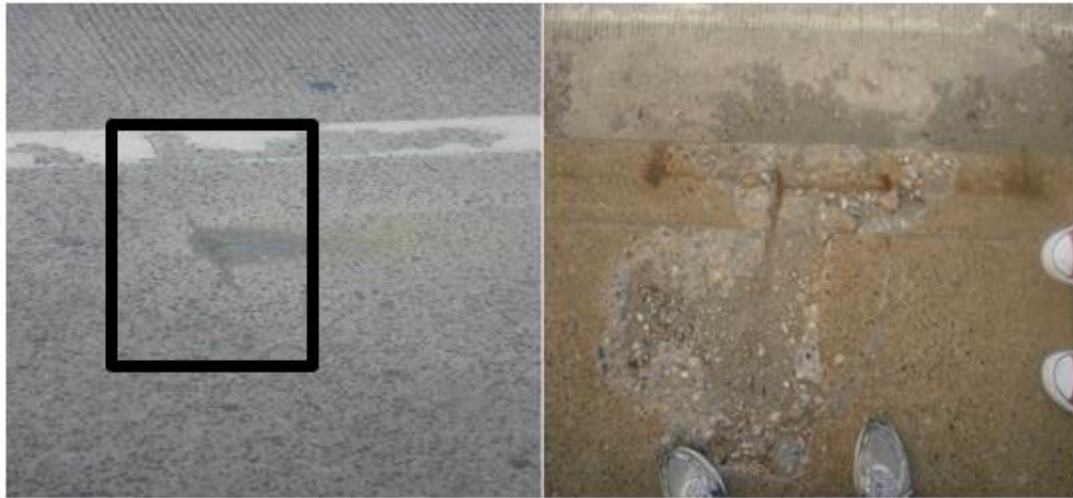
Figure 2.13: Examples of corrosion cracks.
