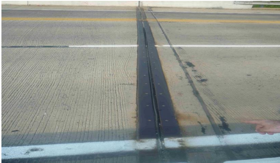
Figure 2.9: Approach slab and joint.
