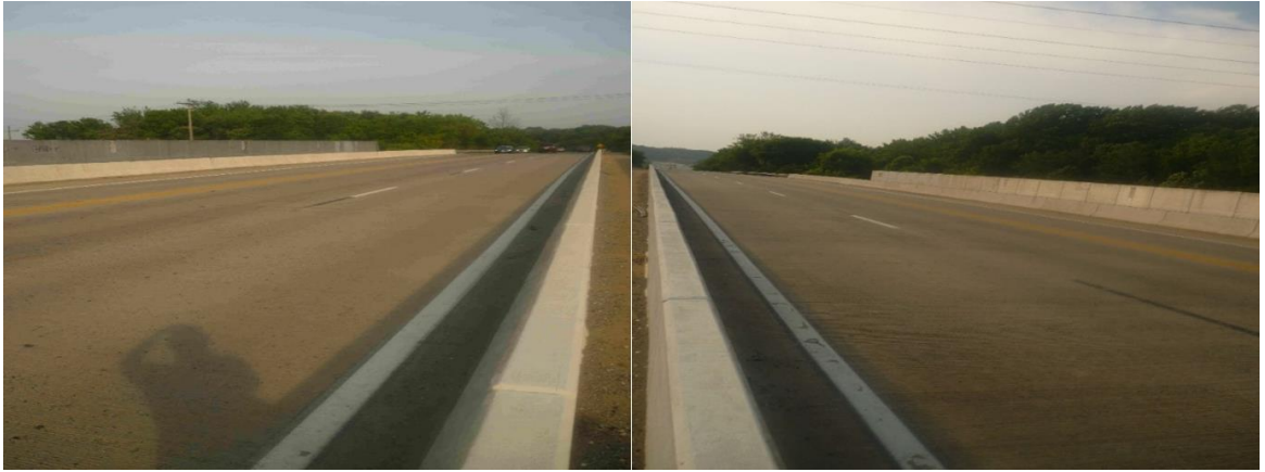
Figure 2.8: Bridge deck from both sides of approaching traffic.
