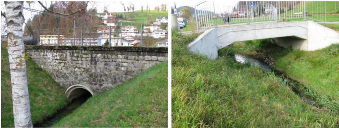
Figure 6.31: Two Examples of Existing Culverts
