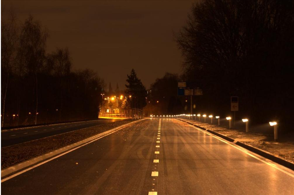
Figure 6.28: Road segment with Low-level Lighting
