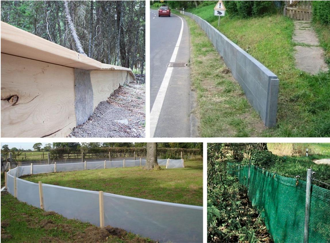
Figure 6.29: Exclusion fences Made of Various Materials
