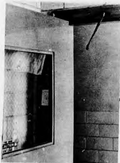
FIRE DOOR on third floor of Colburn will not close when swung open - a violation of fire codes.
