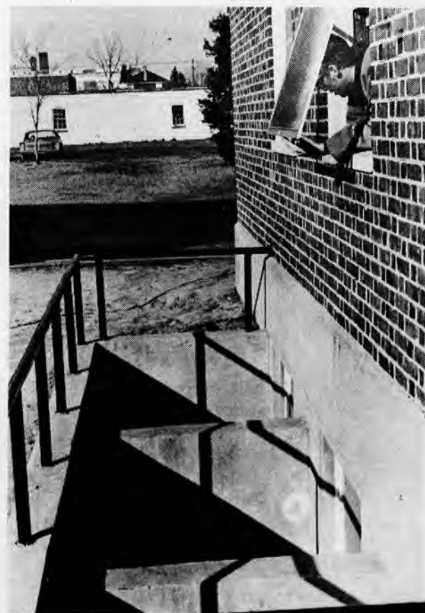
WINDOW WELLS below director's apartment at Colburn provide a hazardous route behind a fire block the only other exit in the apartment.
