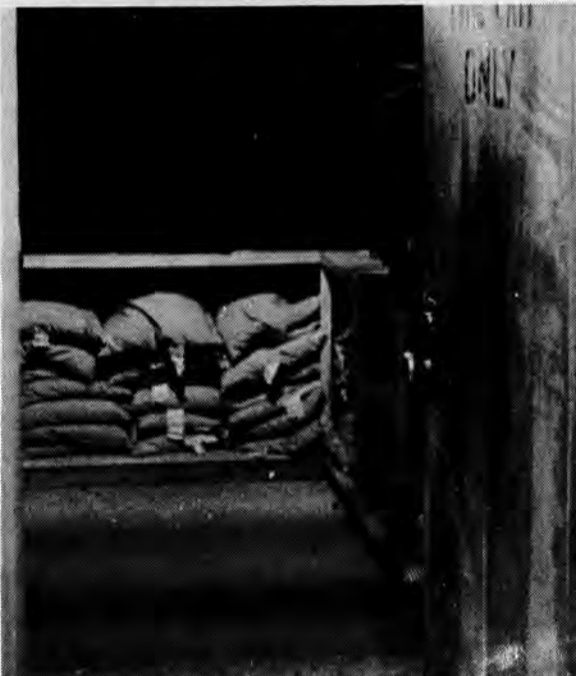
...it reveals a room with no exit, thus making the door marking hazardous in event of a fire.
