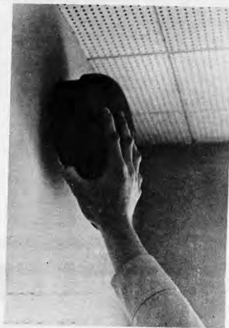
FIRE BELL on second floor of Colburn can be spun causing a weakring should the alarm system be activated.
