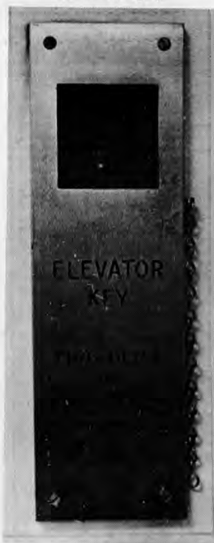
ELEVATOR KEY in basement of Student Center has been broken and missing for months. The key enables firemen to put the elevator under their use in an emergency situation.
