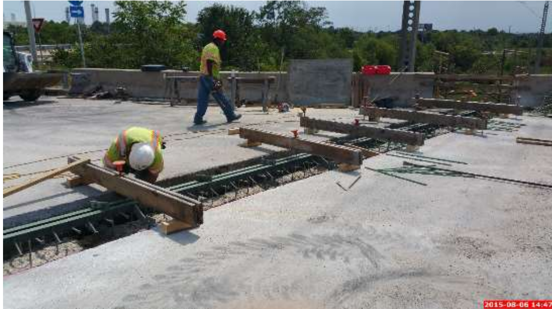
Figure 55: The Temporary Anchorage of the Armoring Systems onto the Deck and Approach Riding Surfaces
