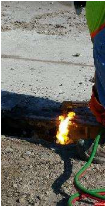
Figure 38 Heat Cutting/Torching of the Armoring
