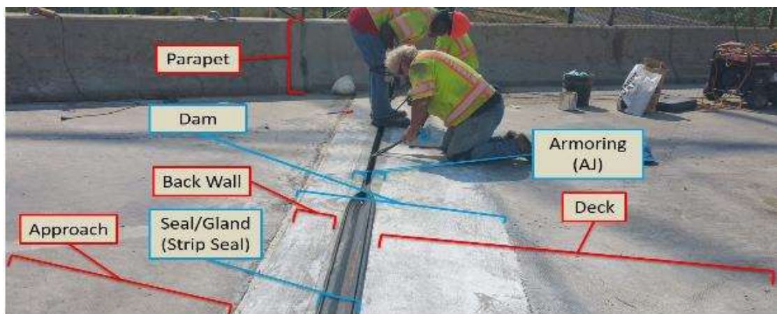
Figure 13: Components Associated with the Replacement of the Southern Abutment Joint Post-Construction
