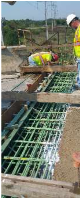
Figure 66 Spraying of the Adhesive Spray
