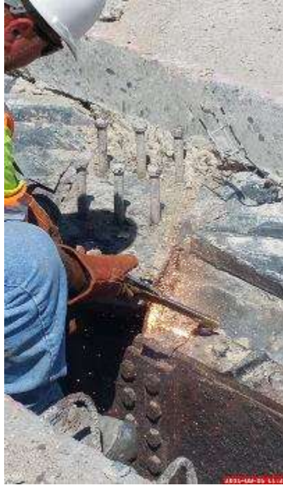
Figure 41: Torching and Removal of the Previous Metal Formwork
