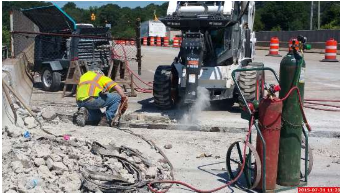
Figure 42: Heat Cutting/Torching Performed Intermittently as Soon as Armoring Elements Made Available to Foreman
