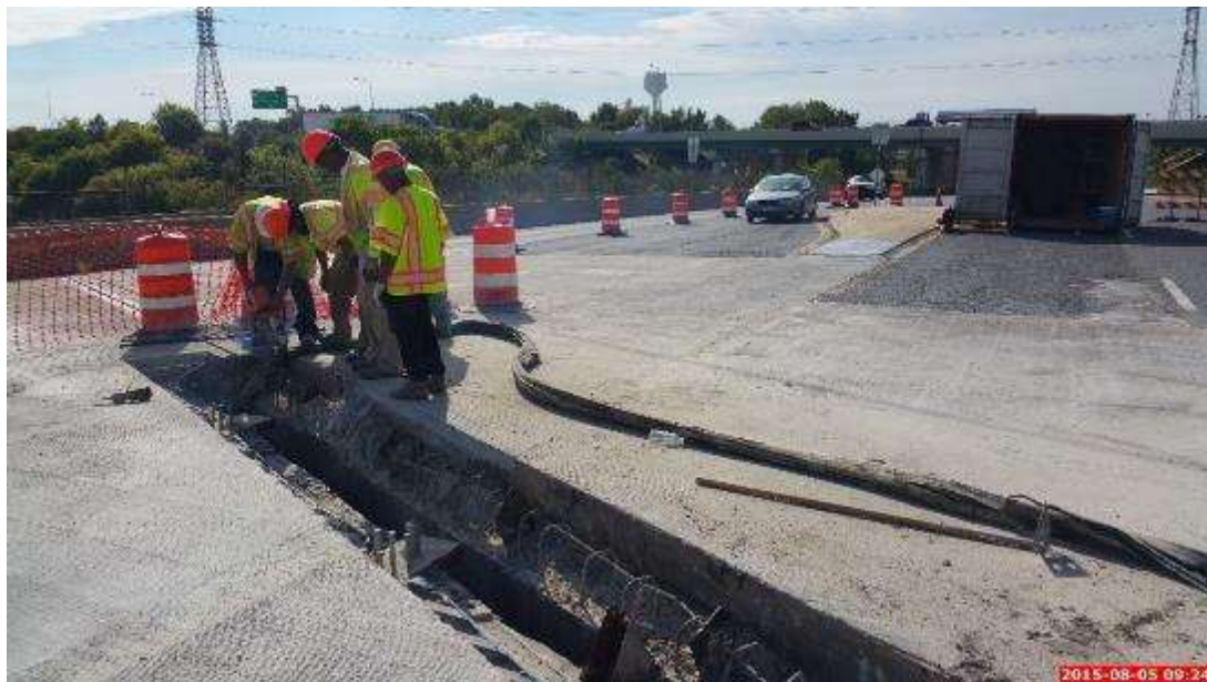
Figure 37: Removal of the Previous Cushion Joint Seal
