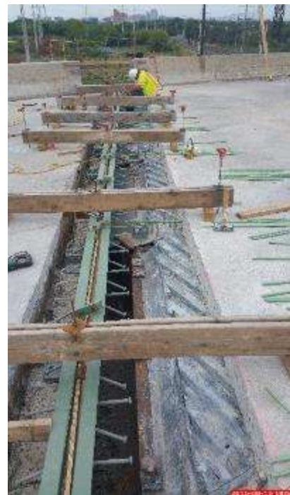
Figure 36 Depiction of the Deck Header (5) and Backwall Anchorage (10)
