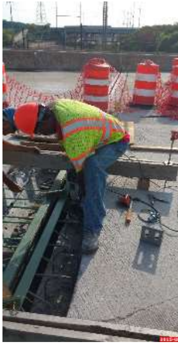
Figure 61 Drilling of the Anchorage Holes in the Backwall
