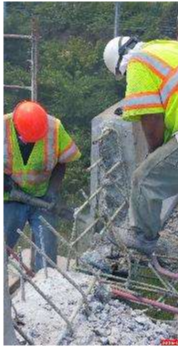
Figure 30 Demolition of the Parapet with a Clear Depiction of the Overhang since the Deck Pan was Punctured by the Skid Steer Loader
