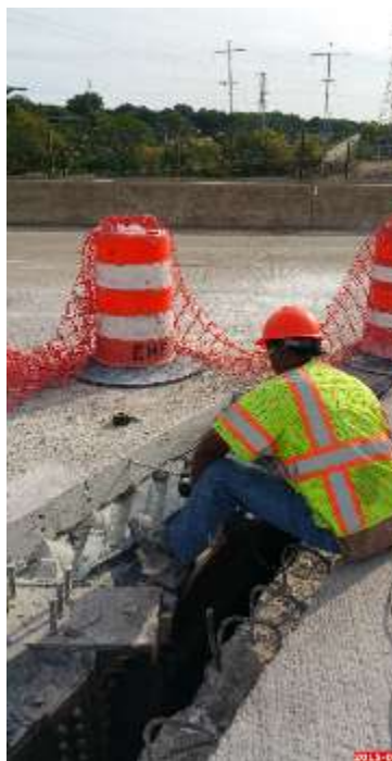
Figure 50 Drilling of the holes for the Dowels
