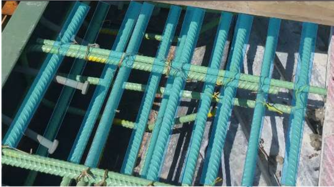
Figure 49: Highlighted in Blue are the Rebars, that are Visible, Running Laterally Along the Demolition Length of the Dam
