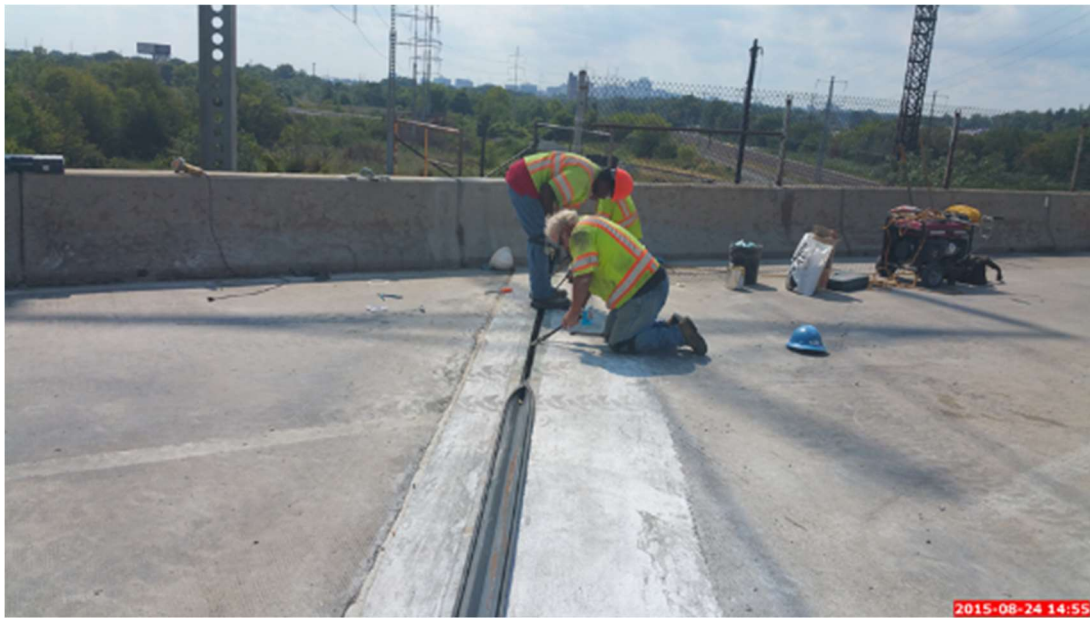
Figure 76: Implementation of the Strip Seal Extrusion into the Armoring
