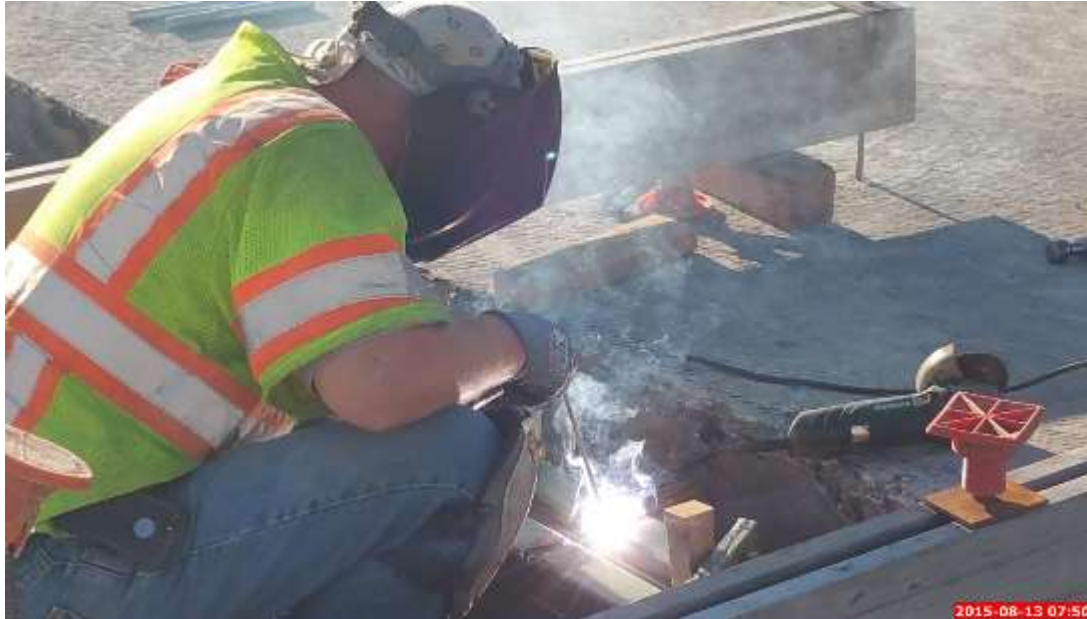
Figure 60: Welding of the Two Separately Delivered and Implemented Armoring Systems to One Another
