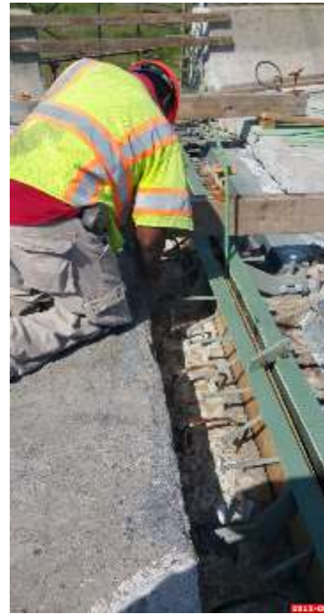
Figure 63 Placement of the Anchorage Component into the Holes with Grout
