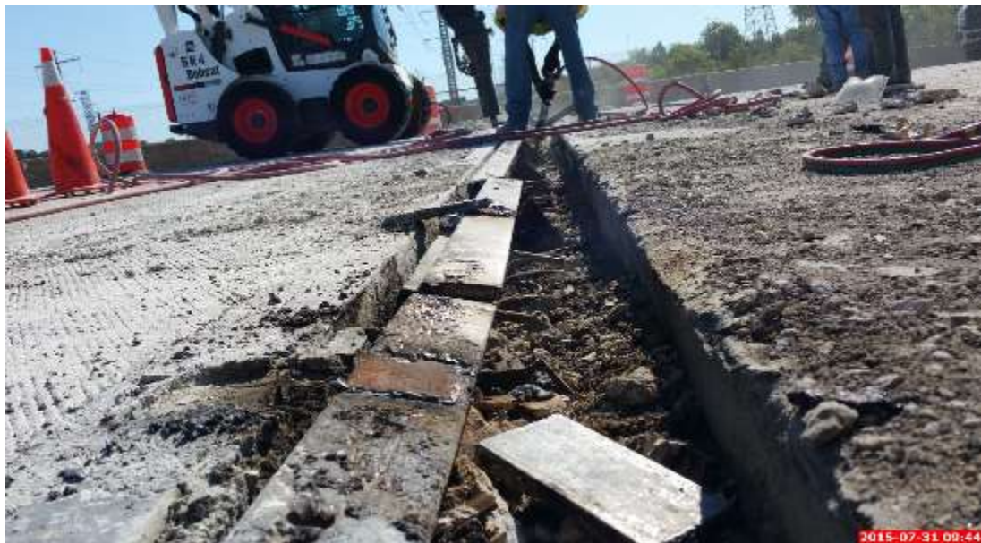
Figure 43: The Skid Steer Loader Breaking on the Deck Header While 30-Pound Breakers Are Utilized on the Backwall
