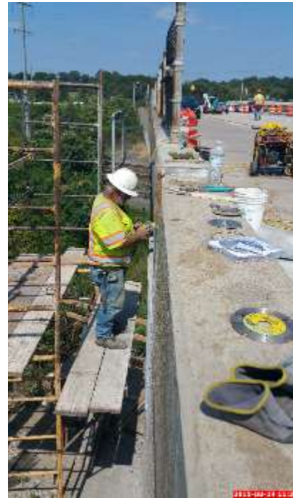
Figure 81 Grinding of Cured Concrete on Parapet Base Fascia
