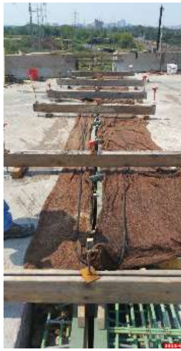
Figure 70 Placement of the Moist Burlap and Weeper Hose
