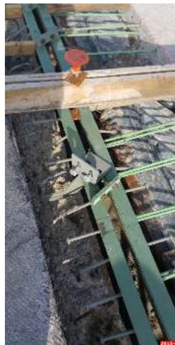
Figure 52 Placement of the Dowels After the Implementation of the New Armoring System
