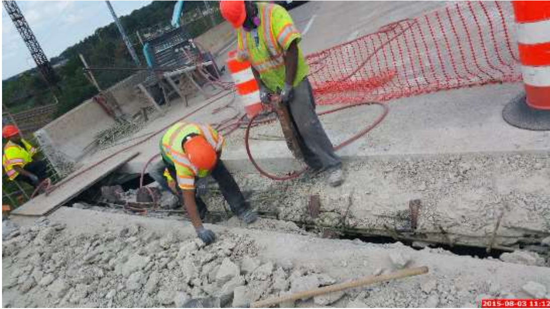
Figure 44: Usage of the 30 Pound Pneumatic Breakers on the Deck Header After Breaking with the Skid Steer Loader Ended
