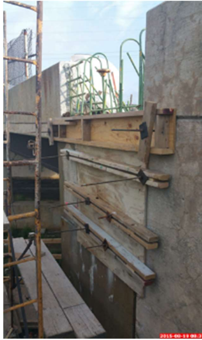
Figure 72: Formwork of the Wing Wall and Parapet Base
