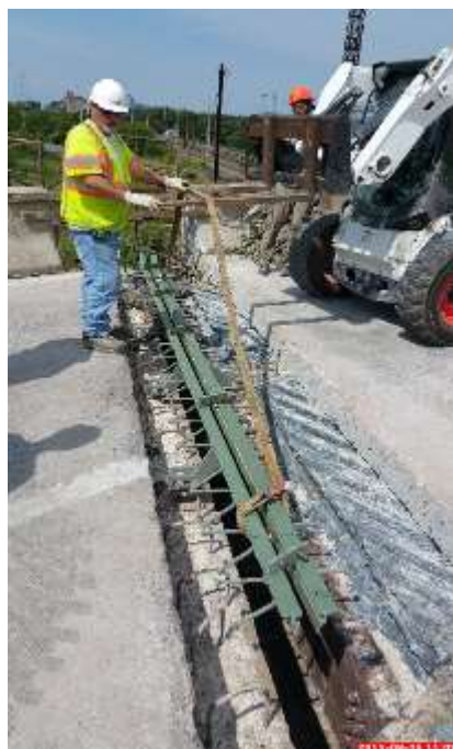
Figure 53 Placement of the Armoring System in the Dam Via Skidder
