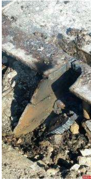
Figure 39 Segmented Armoring, (with Torch), Momentarily to be Detached when Banged with Breaker
