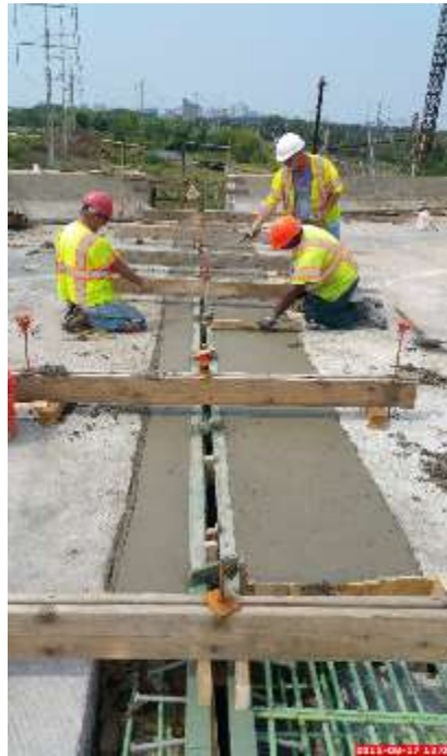
Figure 47: Length Difference Between Pouring and Demolition, the Concrete Held in Place by the “Bulkheads”
