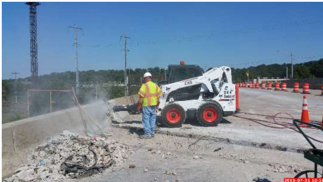
Figure 45: Parapet Body Subjected to Breaking from Skid-Steer-Loader
