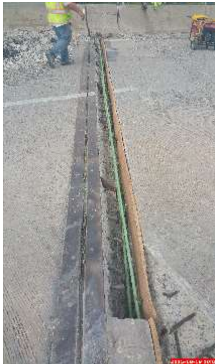
Figure 20: Shallow Depth Removal of North Abutment Backwall Expansion Joint, with Partial Deck Patching in the Surrounding Area
