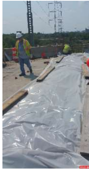
Figure 71 Placement of the Plastic Tarp atop of the Wet Burlap and Weeper Hose
