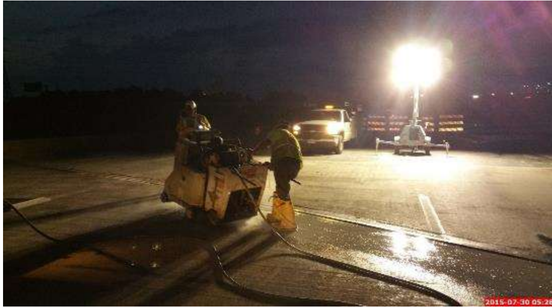
Figure 32: Pre-Construction, Deck Header Segmentation Through Concrete Saw Cutting with the Walk-Behind-Saw
