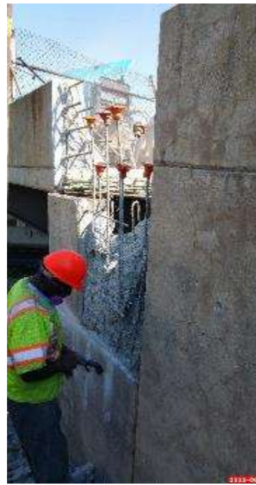
Figure 31 The Completion of the Parapet and Wing Wall Demolition
