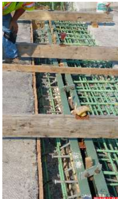
Figure 65: The Cork Formwork Can Be Seen Along the Backwall-Approach Riding Surface Interface, Parallel to the Newly Implemented Rebars
