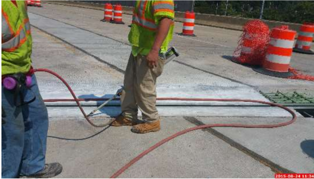
Figure 75: Application of Silicone Within the Backwall and Approach Riding Surface Interface, Above the Cork Formwork
