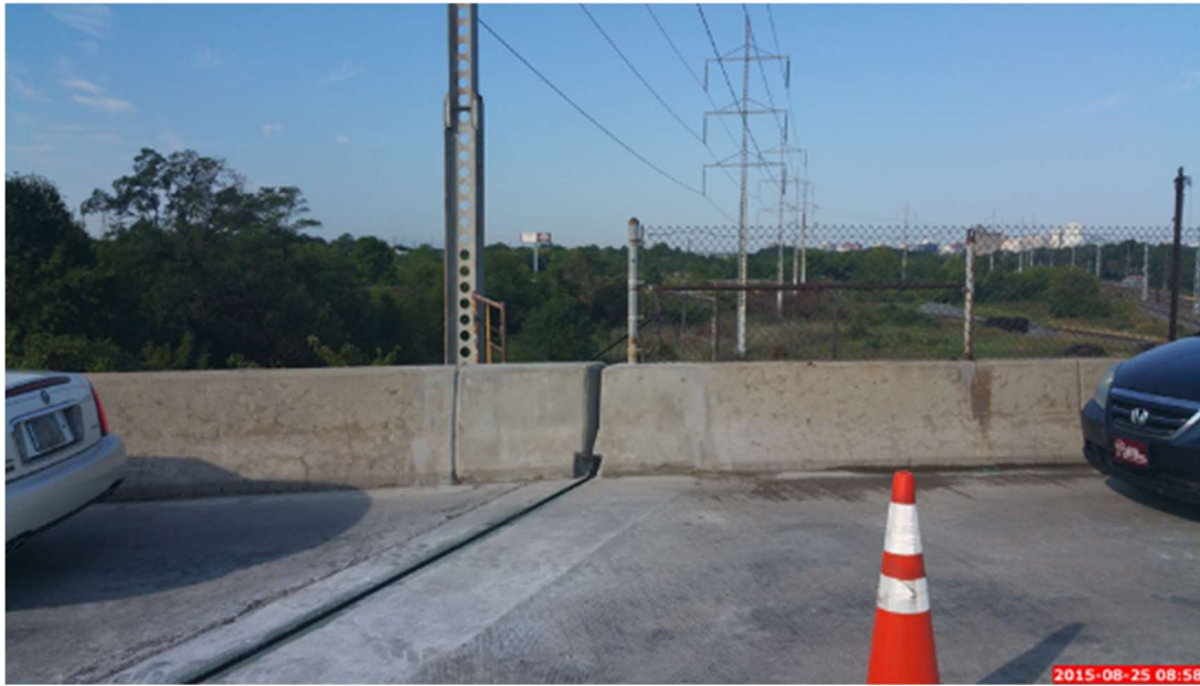
Figure 77: Depiction of Replaced Headers of Lane 1 and the Parapet Resulting from Completion of the Case-Study
