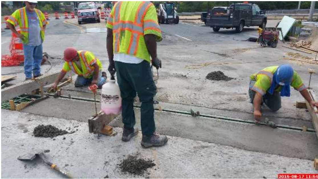
Figure 68: The Smoothing of the Newly Poured Concrete Paired with the Spraying of the Curing Compound
