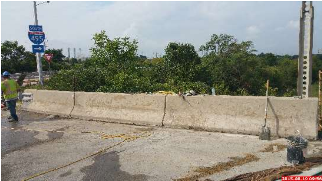
Figure 22: The region of backer rod and silicone between the parapet to approach and backwall header interface to be implemented
