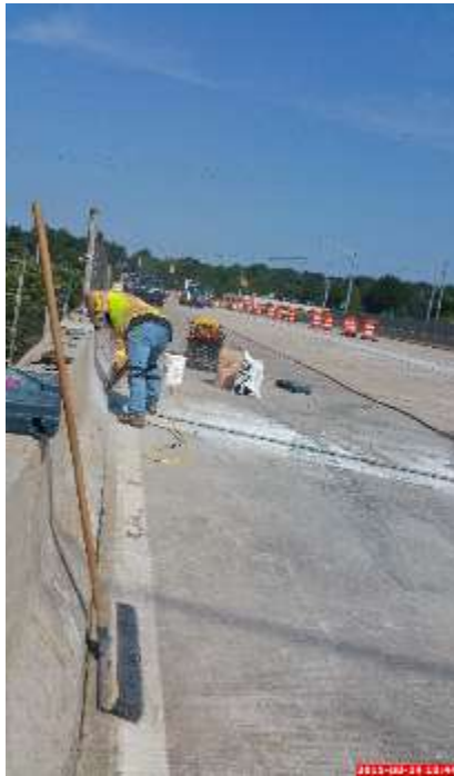
Figure 80 Grinding of Cured Concrete on Roadway Parapet Face
