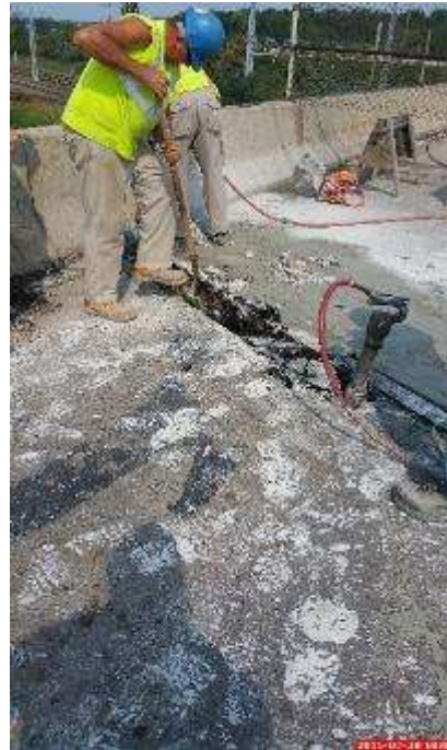
Figure 34 Depiction of the Malleability of the Backwall Header (HMA) Excavated through the Use of a Shovel
