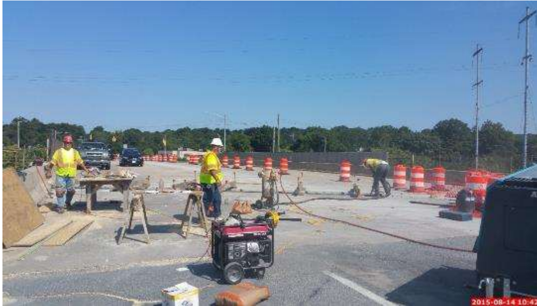
Figure 79: An Example of an Intermittent Sandblasting Session in the Dam In- Between the Placement of the Rebars in the Deck and Backwall Headers
