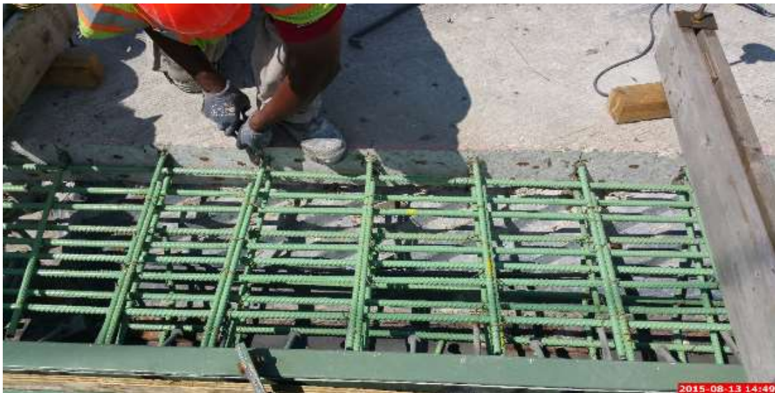
Figure 64: Implementation of the Stirrups and Rebars Through Tying
