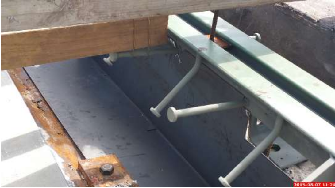
Figure 59: The Metal Formwork Running Along the Pouring Length of the Dam, Connected to the Diaphragm and Bottom Lip of the Armoring
