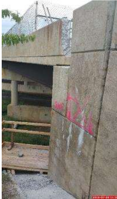
Figure 14: Wingwall, indicated by the Spray-Paint, to be demolished
