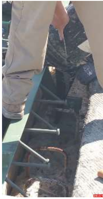
Figure 62 Pouring of Grout in the Anchorage Holes
