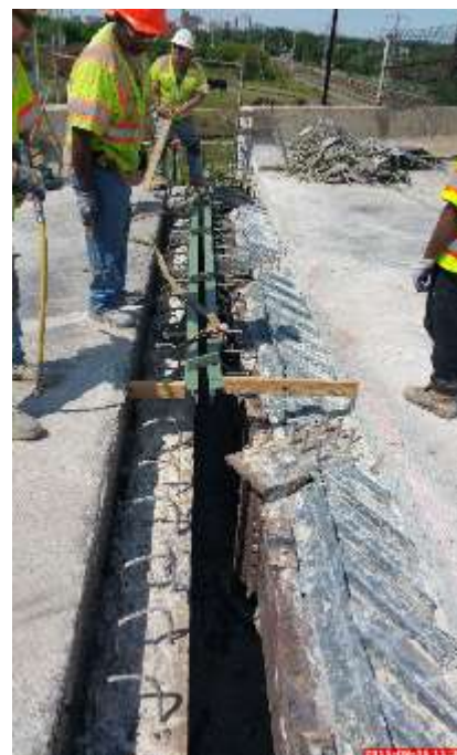
Figure 54 Adjustment of the Armoring System in Dam by Hand
