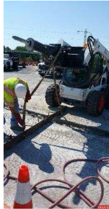
Figure 40 Removal of Armoring with Skid Steer Loader
