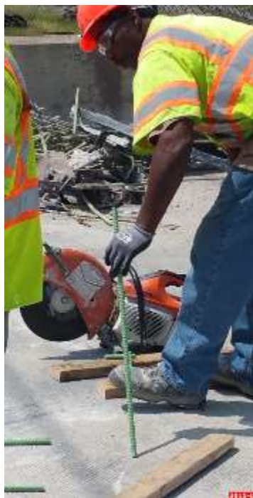
Figure 51 Adjusting the Length of the Dowels to Fit the Holes
