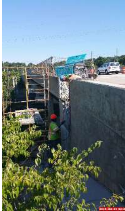
Figure 46: Wing Wall, and the Parapet Base Subjected to Breaking from the Thirty Pound Breaker
