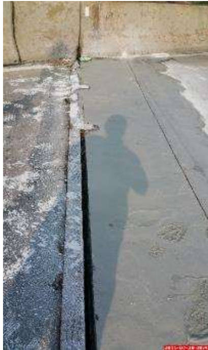
Figure 33 The Dam Post-Concrete Saw Cutting and Pre-Construction. Notice the Welded Plates on the Armoring and the HMA
