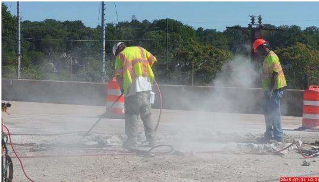
Figure 78: An Example of One of the Many Intermittent Airblasting Session at the End of the First Day of the Demolition Stage
