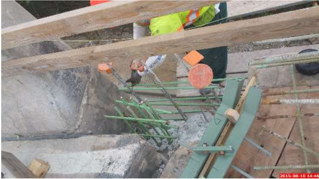
Figure 56: The Intermittent Placement of the Wing Wall/ Backwall Sided Parapet Base Steel Reinforcement
