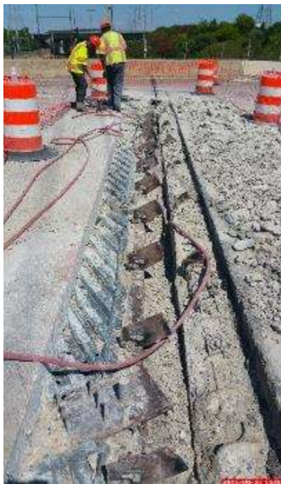
Figure 35 Depiction of Deck Header (10) and Backwall (5)
