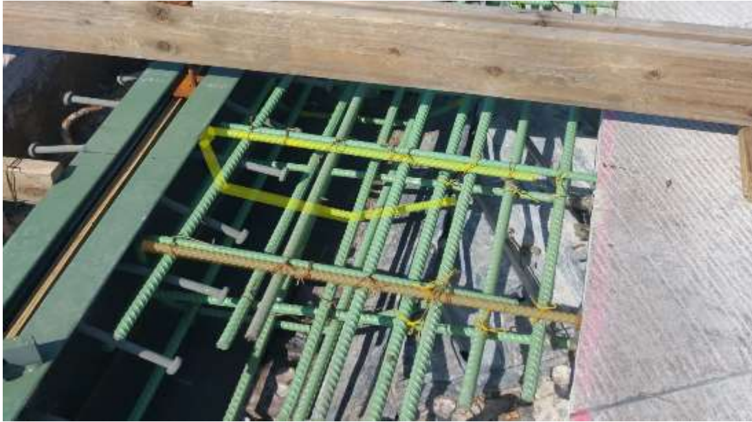
Figure 48: Highlighted in Orange is a Dowel Epoxied into the Deck Wall; Highlighted in Yellow is a Stirrup Tied to its Corresponding Dowel.
