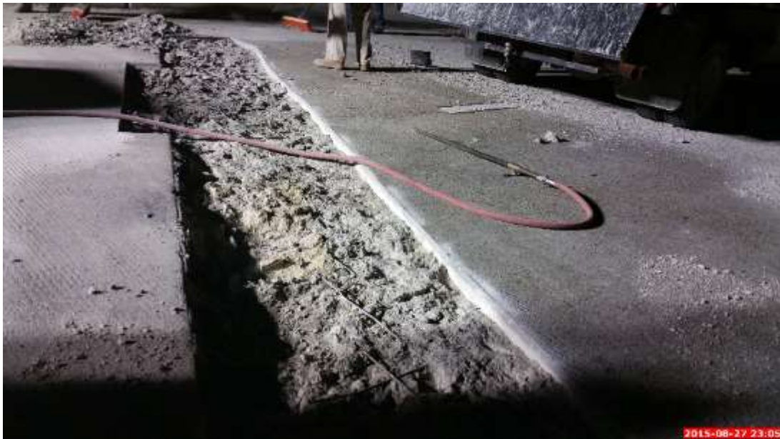
Figure 21: A deck Patching Operation that Provided a Shallow Depth Concrete Replacement to the Upper Steel Reinforcement Mat
