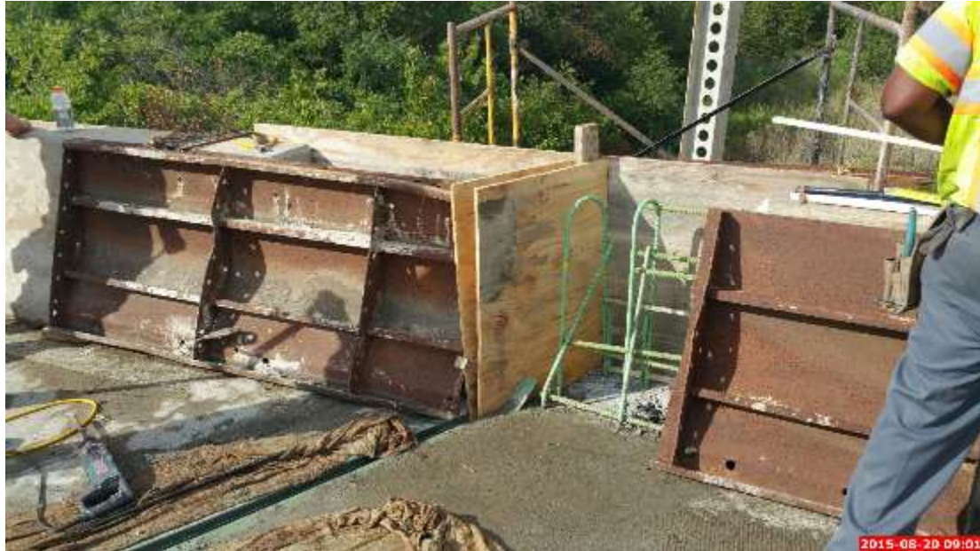
Figure 74: Formwork of the Parapet Bodies
