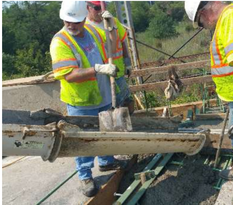
Figure 67 Pouring of the Concrete from the Truck, assisted with a Worker with a Shovel, with a Mechanical Vibrator Placed Within the Newly Poured Concrete to Facilitate Dissemination of the Concrete
