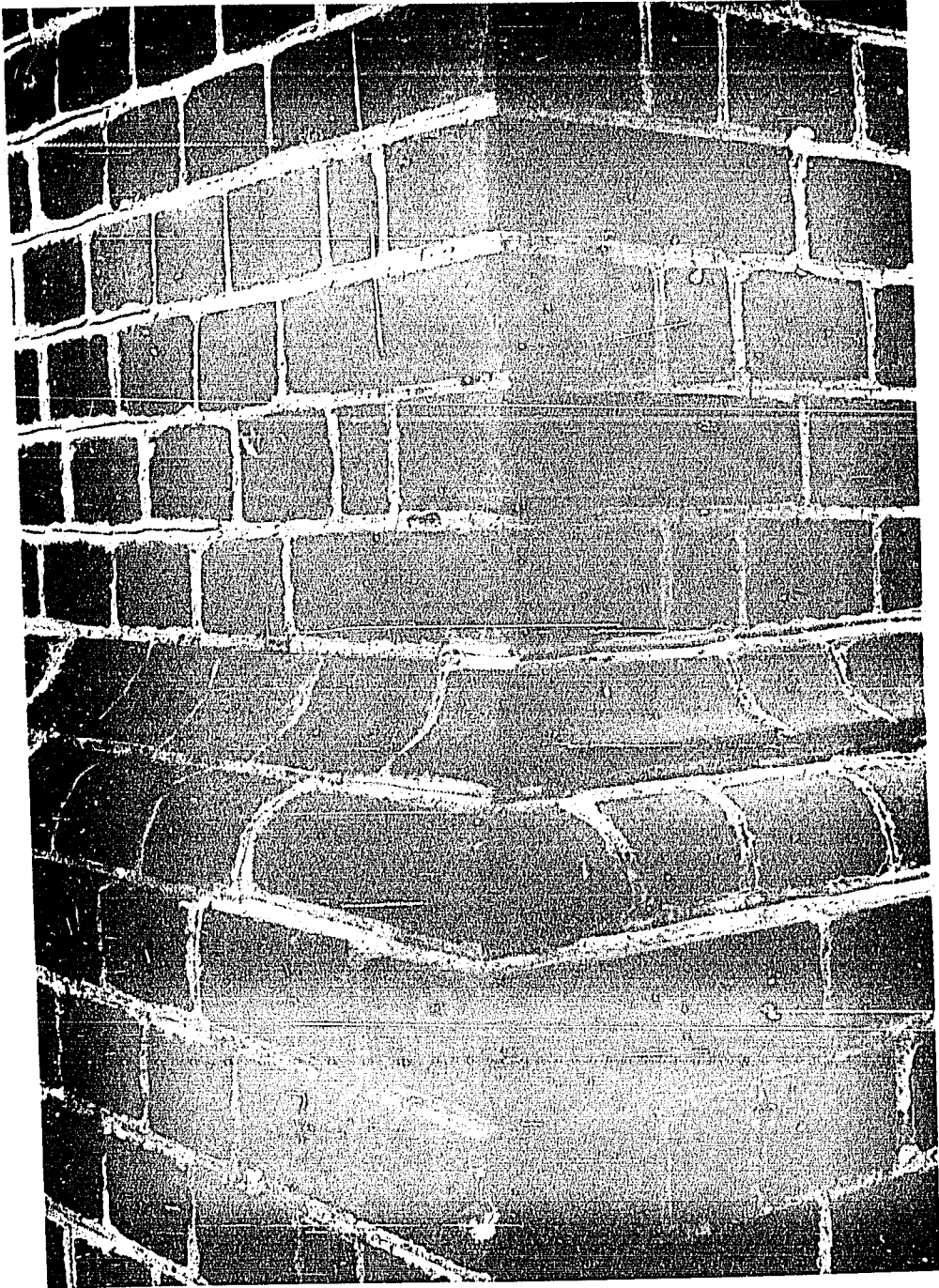
The double course of molded bricks, which cap the raised watertable, is one example of the finely executed exterior masonry.
