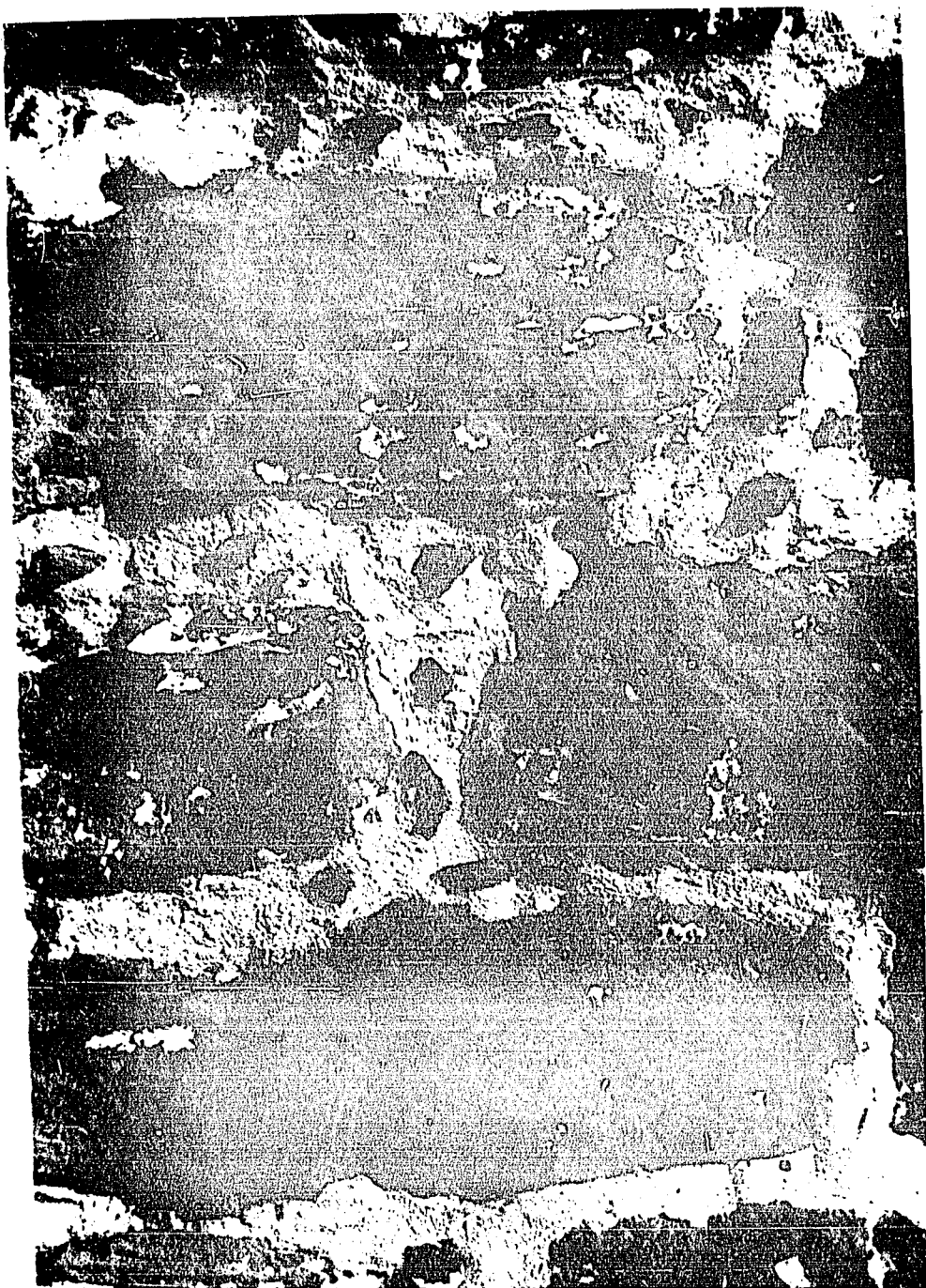
A detail of the galleting from "Handcock's Resolution," a planter's house from the 1760s in northern Anne Arundel County.
