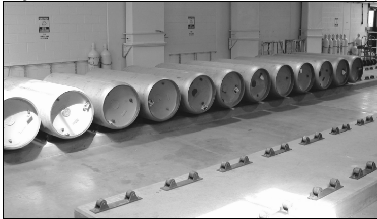
Figure 5. Chlorine canisters at a wastewater treatment facility 62
