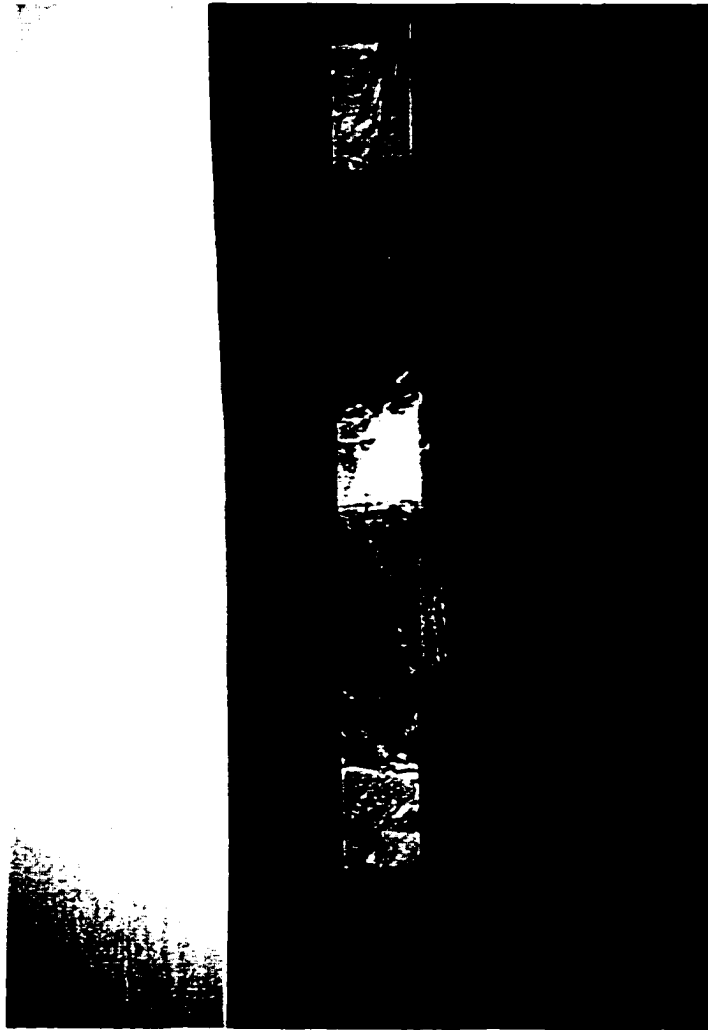
Figure 27. Space between the interior wall of the Gates House and the exterior wall of the Golden Plough Tavern. The plaster wall is the Gates House and the log wall is the Plough Tavern. Courtesy, The York County Heritage Trust, PA.
