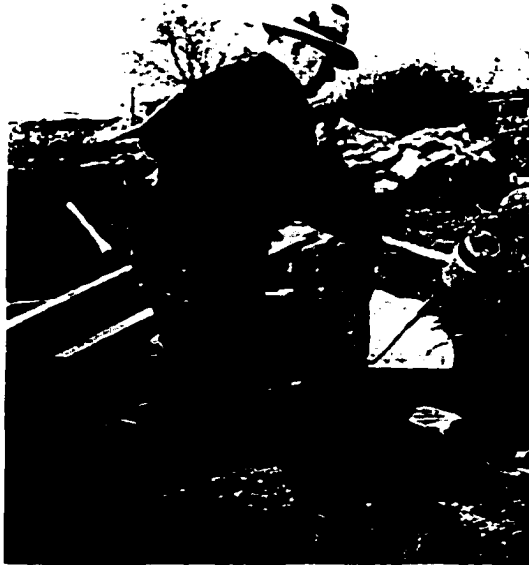
Figure 11. The first step in making clapboards: splitting the log. Ephrata, mid-1940s. Courtesy, The Winterthur Library: Joseph Downs Collection of Manuscripts and Printed Ephemera, No. 84x76.
