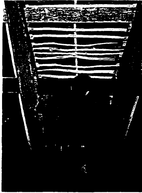
Figure 23. Restoring wattle and daub in the Golden Plough Tavern, 1961-1964. Courtesy, The Winterthur Library: Joseph Downs Collection of Manuscripts and Printed Ephemera, No. 84x76.
